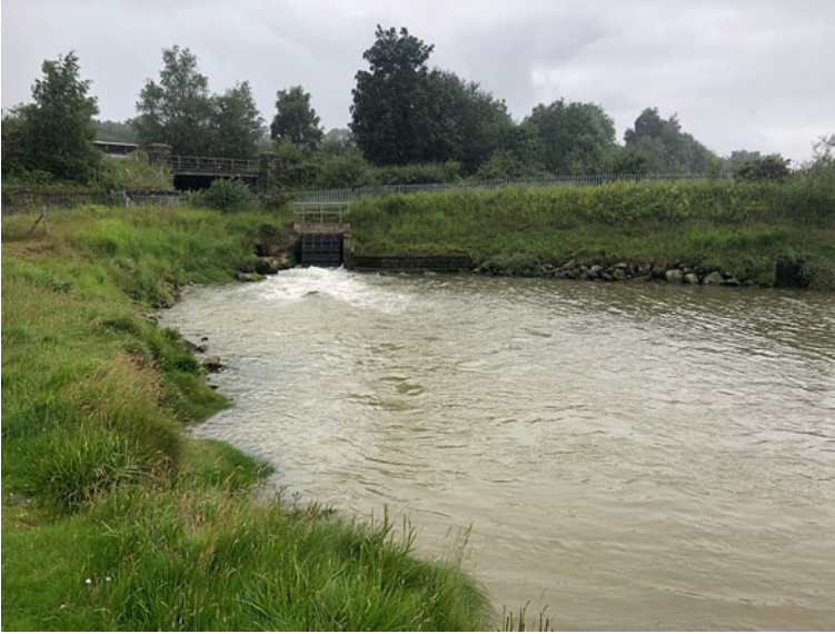
Fig. 3 The Milwr Tunnel outfall into the Dee Estuary, near Bagillt, Flintshire. Photograph: Mark Nuttall
