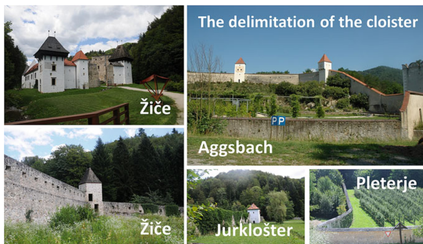
Fig. 7 The enclosure wall
