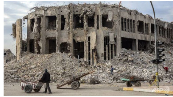
Fig. 8 The remaining three floors of The Insurance Building after demolition, demolished later. Source Website N(7)
