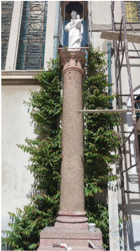
Fig. 20 The granite column next to the church's entrance (photographed by the author)
