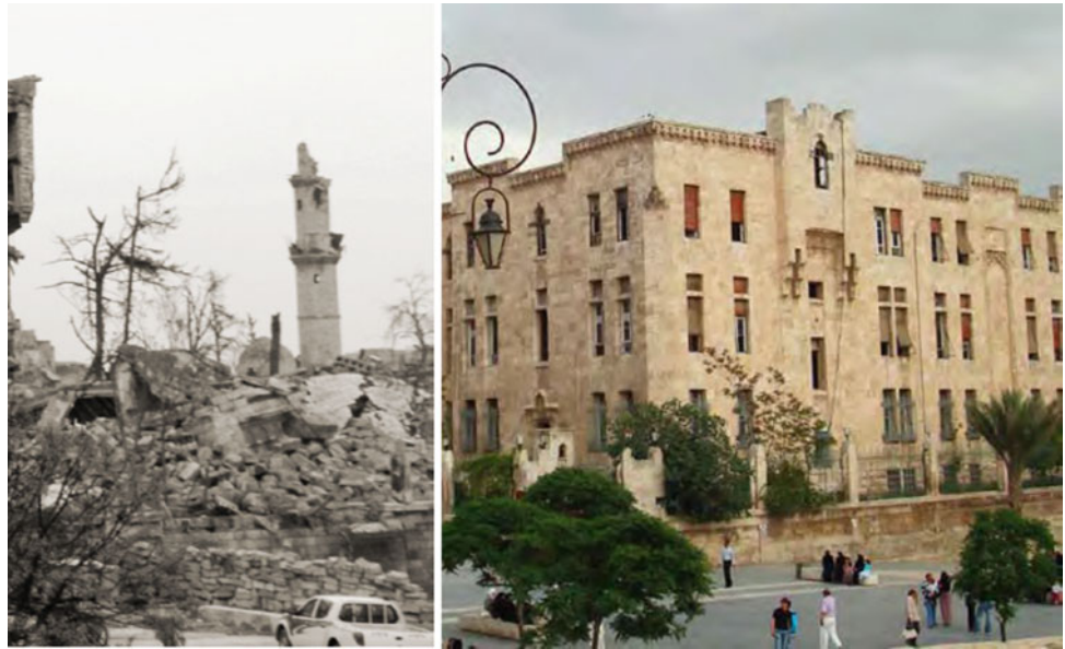
Fig. 15 Extent of damage to the Grand Serail government building (left) and how it looks before the damage (right) (UNESCO, 2017)
