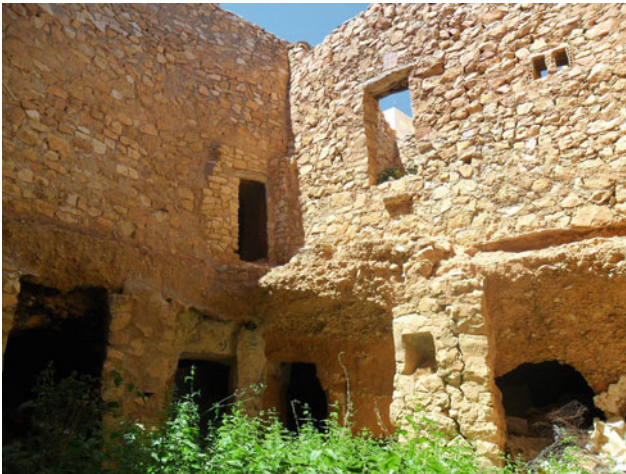
Fig. 7.14 Built spaces in a cave dwelling (Author's photos)
