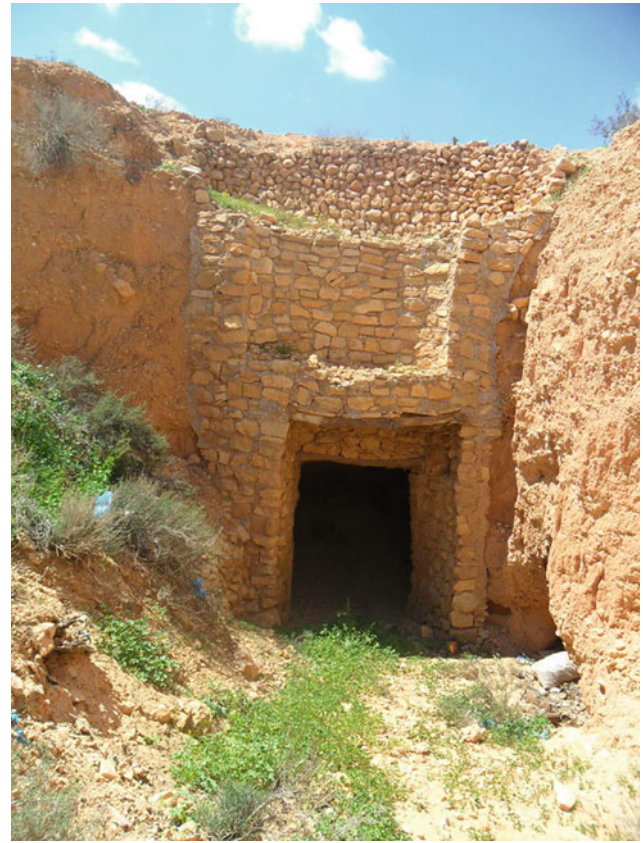
Fig. 7.12 The reinforcement of an entry by a stone apparatus (Author's photos)
