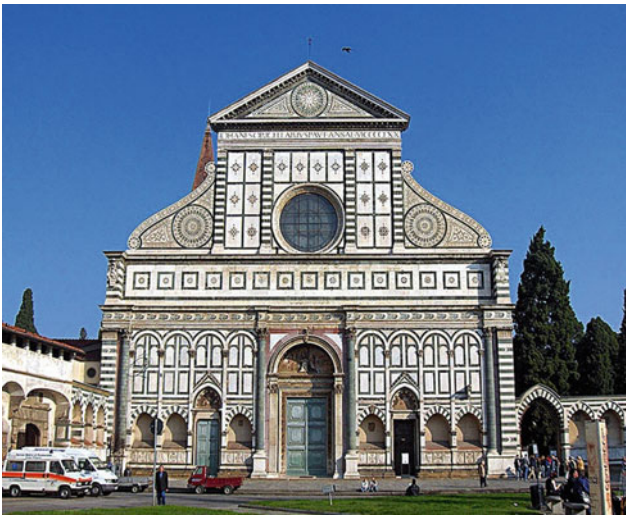
Fig. 5 Façade of Santa Maria Novella, a church in Florence, Italy, by Leon Battista Alberti 1420–1470 (Beniscelli & Furlan, 2005)
