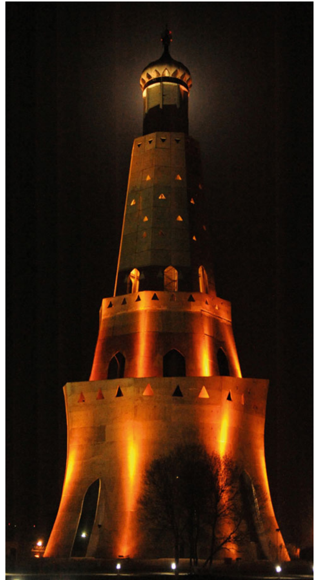
Fig. 11 Colour wash lights on Fateh Burj
