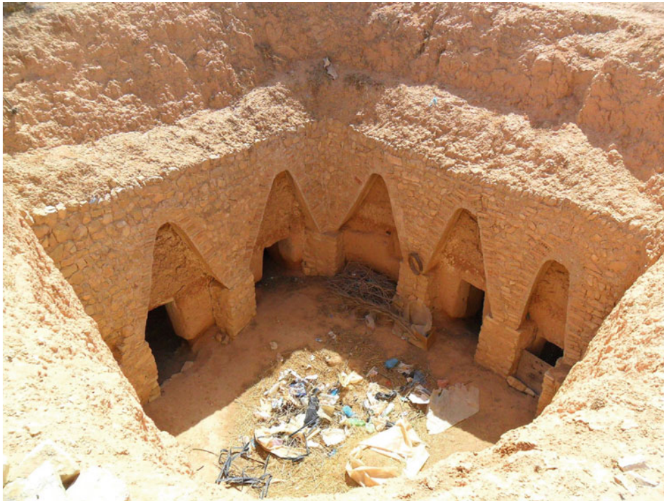
Fig. 13 The reinforcement of patio walls by a stone and brick apparatus (Author's photos)
