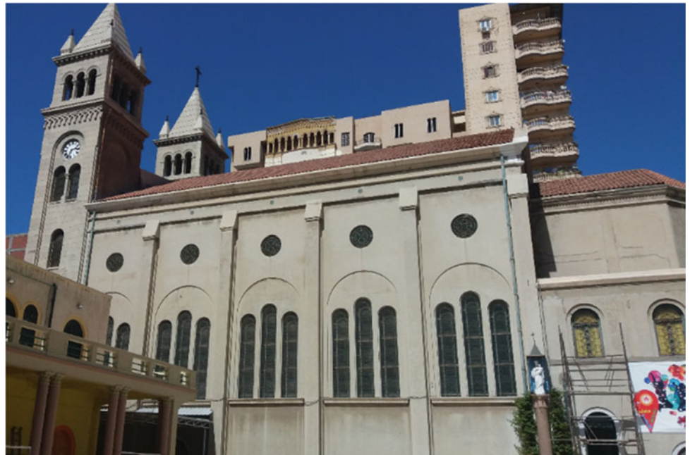
Fig. 6 The side façade that has the current entrance of the church (photographed by the author)
