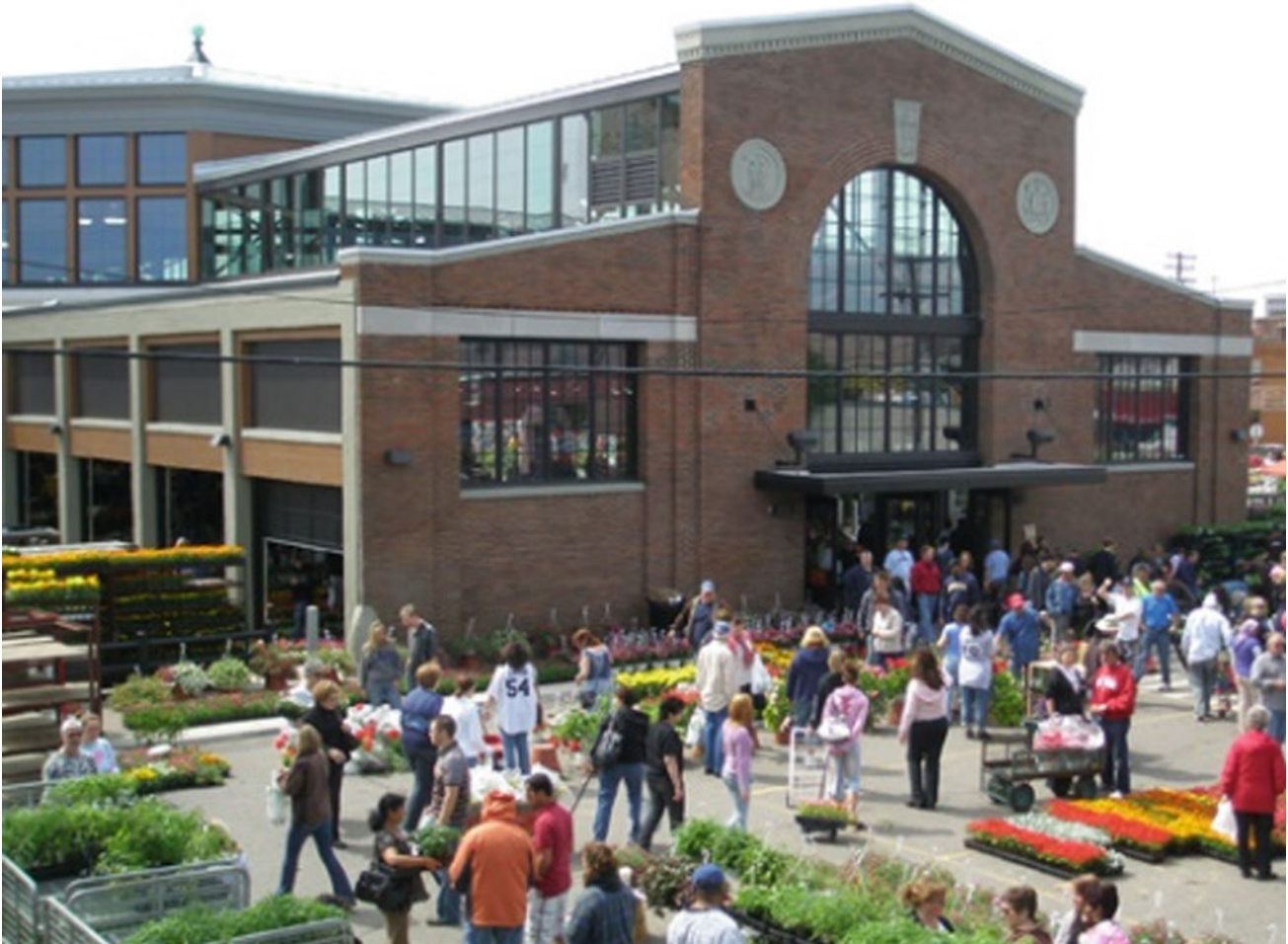
Fig. 8 Renovated Shed 3 historic market in Detroit. Source Eastern Market Corporation (2018)
