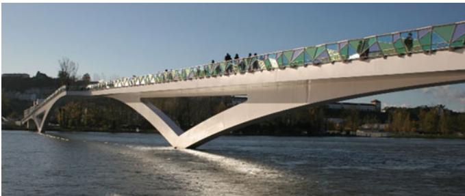
Fig. 4 Coimbra footbridge: lateral view
