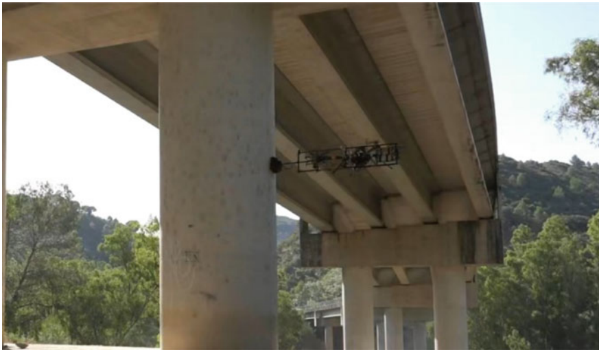
Fig. 2 Bridge contact inspection aerial robot
