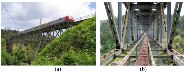
Fig. 14 Trezói bridge: a lateral view; b view inside the deck
