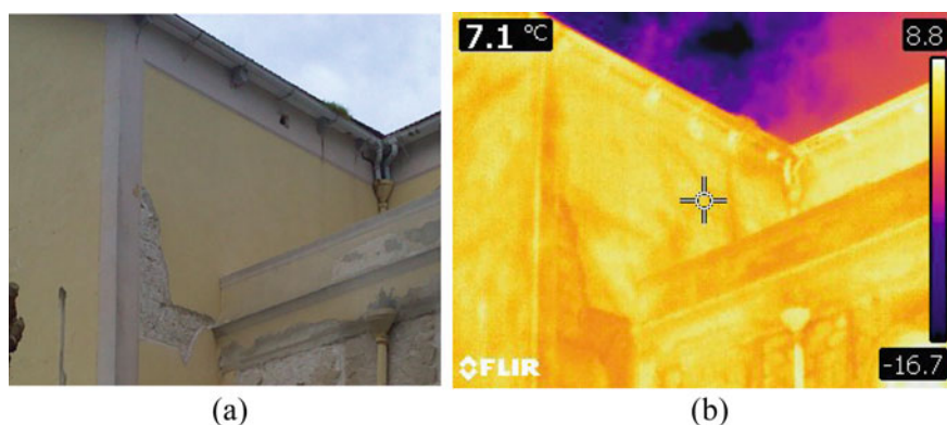
Fig. 6 Thermographic survey of the transept from the ground floor
