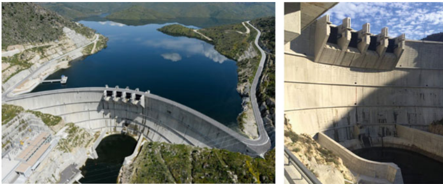
Fig. 34 Baixo Sabor arch dam, aerial view of dam and reservoir and detail of the spillway from downstream [51]
