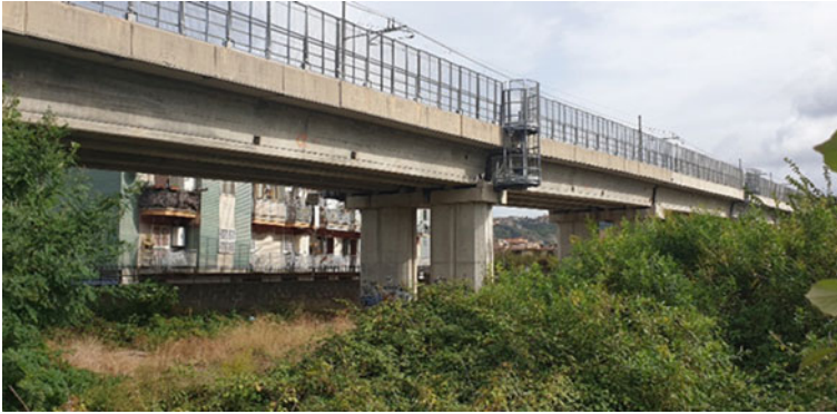
Fig. 4 View of the bridge near to Quarto Stazione (P29)
