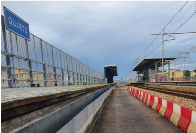
Fig. 5 View of Quarto Station from top of P39 on railway #2 (no installations)
