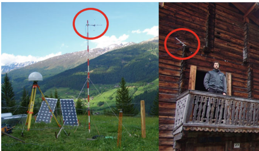
Fig. 5 Continuous measurements with data transfer over radio link, left: radio antenna at a site, right: radio antenna at the calculation center
