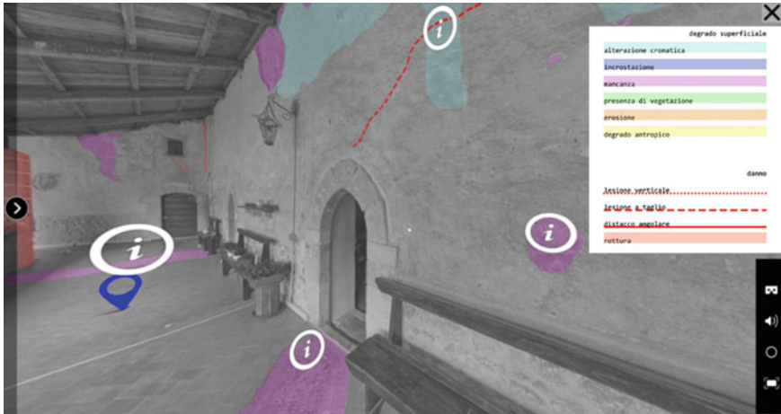
Fig. 6 Virtual tour of the damage path with information hotspots and damage survey legend
