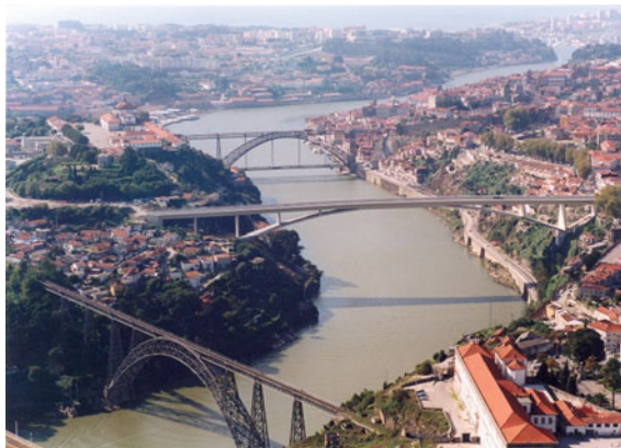
Fig. 17 Aerial view of Maria Pia, Infante D. Henrique and Luiz I bridges (from bottom to top) over Douro river at Porto
