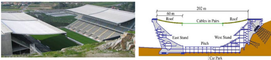
Fig. 24 Braga Municipal Sports Stadium: view of roof from the west side. Cross section
