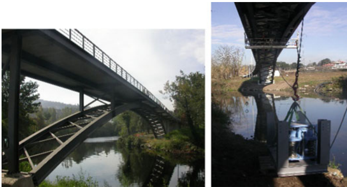
Fig. 1 Santo Tirso footbridge: lateral view (left), installation of a TMD (right)
