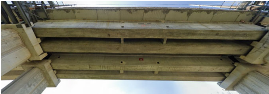
Fig. 3 Picture of a single span of the bridge from below
