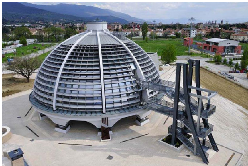
Fig. 1 Monitored operation room building
