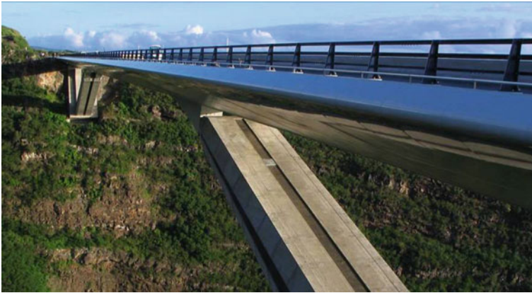
Fig. 22 Grande Ravine viaduct, Reunion Island
