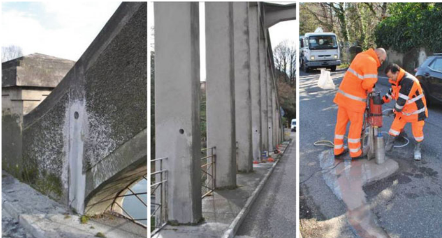
Fig. 6 Coring samples from arches, hangers and deck
