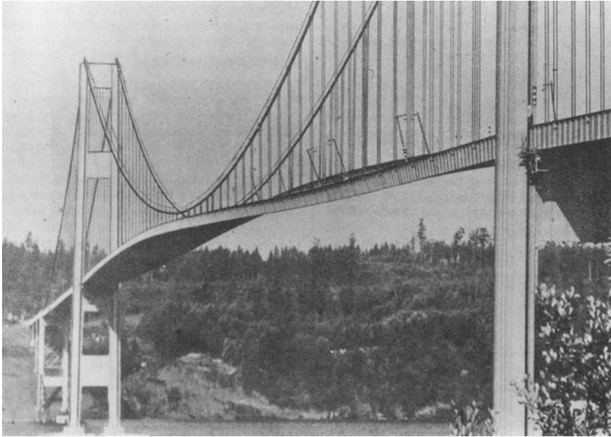
Fig. 2 Flutter of the Tacoma Narrows Bridge, November 10, 1940. From F.B. Farquharson (ed.), Aerodynamic Stability of Suspension Bridges , 1949–1954
