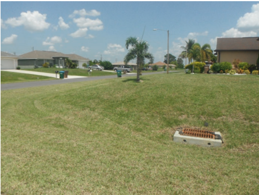
Fig. 12.10 Ground view of water retention basin that was provided during Cape Coral's utilities expansion program. (Source: Photo taken by the author)
