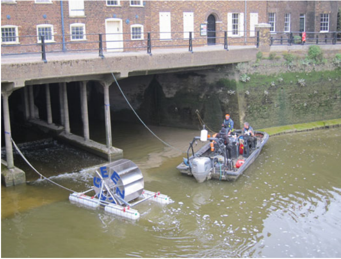
Fig. 5.4 Installation of the water wheel at the Three Mills
