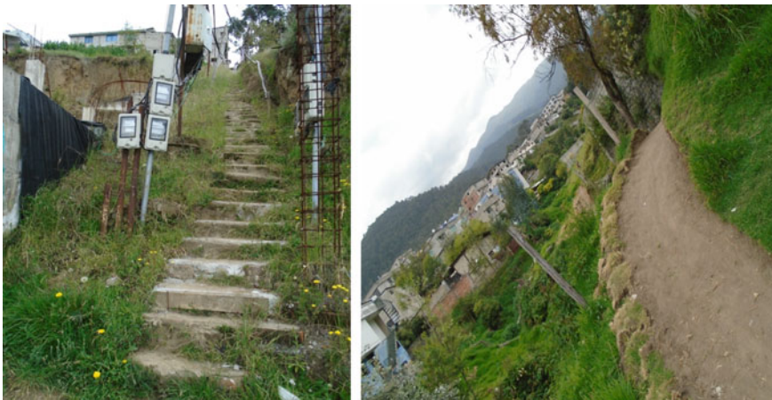
Fig. 8.2 Footpaths and mobility infrastructure in La Pulida (Northwest of Quito)
