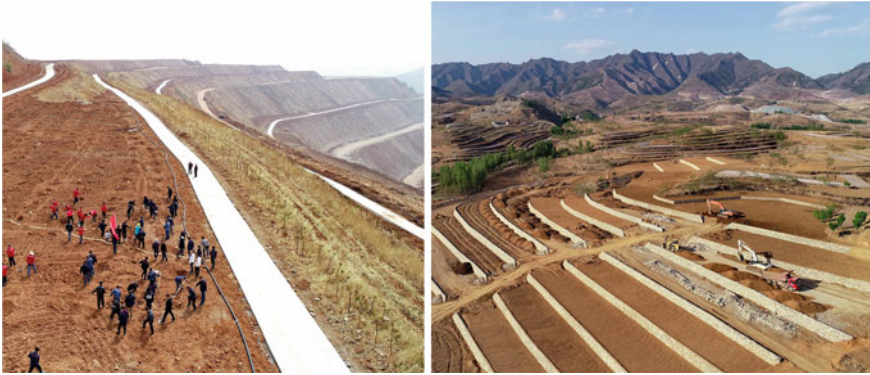
Fig. 9 Diagram of landslide and collapse prevention project. The image demonstrates the retaining wall of soil erosion and slope improvement project in the north and south mountain area. Source Xining Forestry Bureau (2015)
