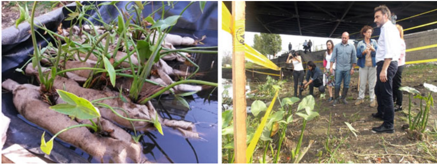
Fig. 6 Revegetation of the riverbanks with native plants. Pictures Ana Faggi
