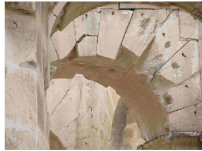
Fig. 2 Archaeoseismological evidence for damaging earthquakes in the middle part of Tunisia. a Dropped arch sectors. El-Djem amphitheatre. #6085. b Extruded blocks. El-Djem amphitheatre. #6062. c Penetrating fracture in arch masonry—parallel to stress. El-Djem amphitheatre. #6098. d Broken corners of columns: axial and oblique. Sousse, Ribat. #5794. Serial numbers refer to images in the archaeoseismological database (Moro and Kázmér 2019). e Shift between column and capital. Sousse, Ribat. #5800. f Twisted walls. Sousse. #5897. g Extruded masonry block. Sousse. #5805. h Displaced arch sector (fallen keystone). Sousse. #5867
