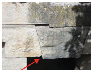
Fig. 2 Damage observed on Algerian Roman sites: a fallen columns in Timgad, b displaced blocks in lintel in Djemila, c displaced block observed in Caracalla Temple in Tebessa
