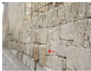
Fig. 2 Damage observed on Algerian Roman sites: a fallen columns in Timgad, b displaced blocks in lintel in Djemila, c displaced block observed in Caracalla Temple in Tebessa
