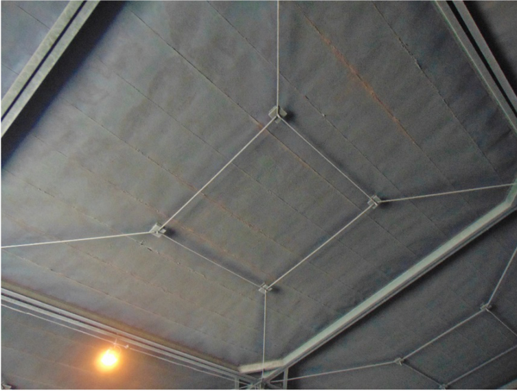
Fig. 2. Steel plate roofing supported by steel ties.
