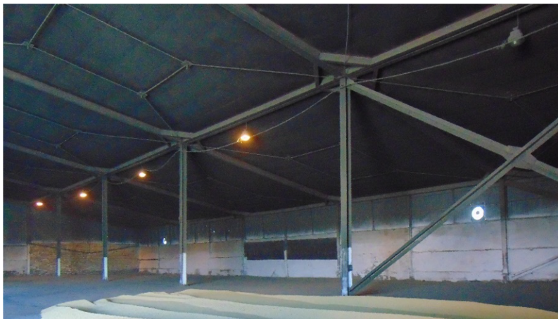
Fig. 1. The frame of the warehouse.
