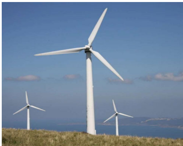
Fig. 3 NEG Micon 1.5 MW Wind Turbine, 68 m diameter Rotor, Tubular Steel Tower. Reproduced from Ref. (Kumar et al. 2018) under Creative Commons license. Copyright @ Gyancity Research Lab (2018)
