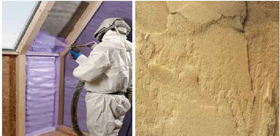
Fig. 3 Foams applied in wall and roof insulation
