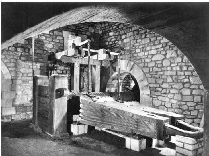
Fig. 12.39 Bellows being recently installed
