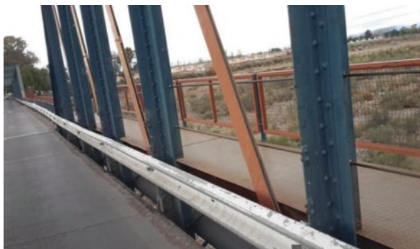
Fig. 12.43 View of the bridge structure consisting of seven sections of 40.6 m
