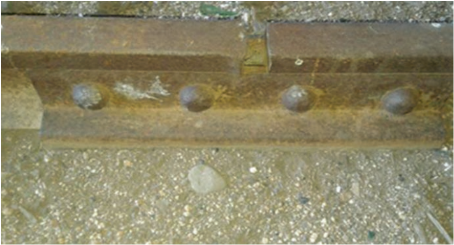
Image 12.23 Function of the threaded bolts is to join rails
