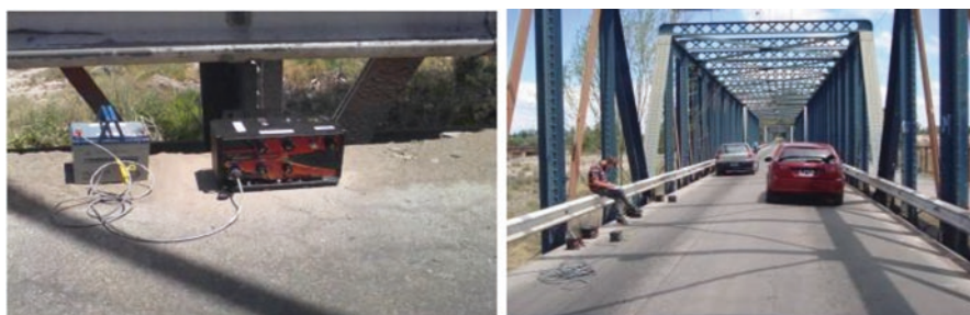
Fig. 12.35 Placement of triaxial accelerometers powered by their corresponding batteries
