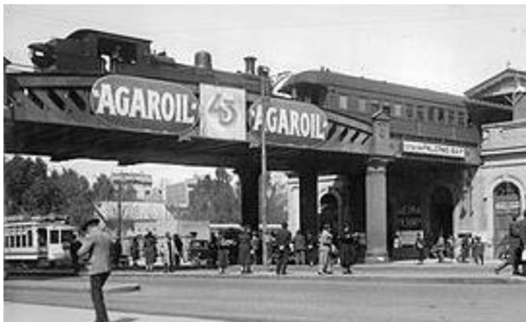
Image 12.9 The emblematic Palermo station in Buenos Aires, Argentina capital city in 1930. Note the inscription “BAP” after the name
