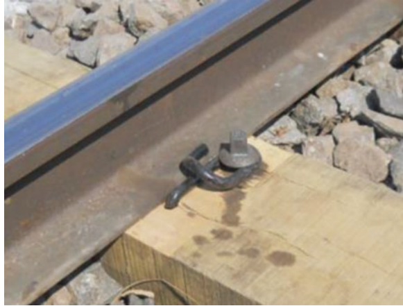
Image 12.12 Gauge-lock (Pandrol clip)
