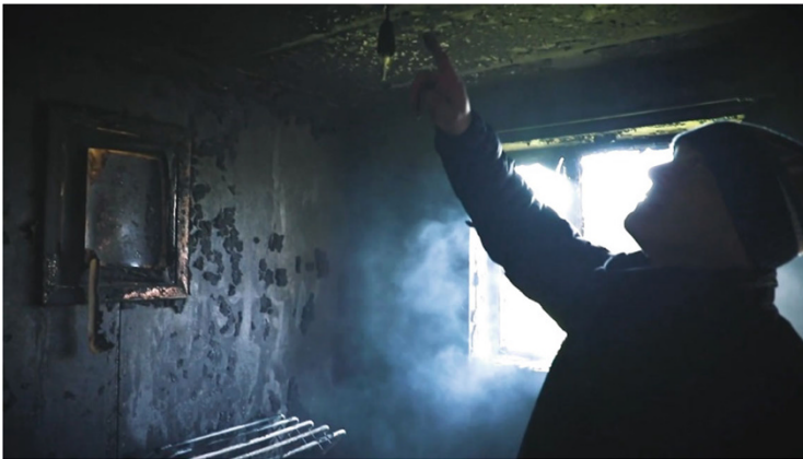
Fire Investigator examining a RiVR scene
