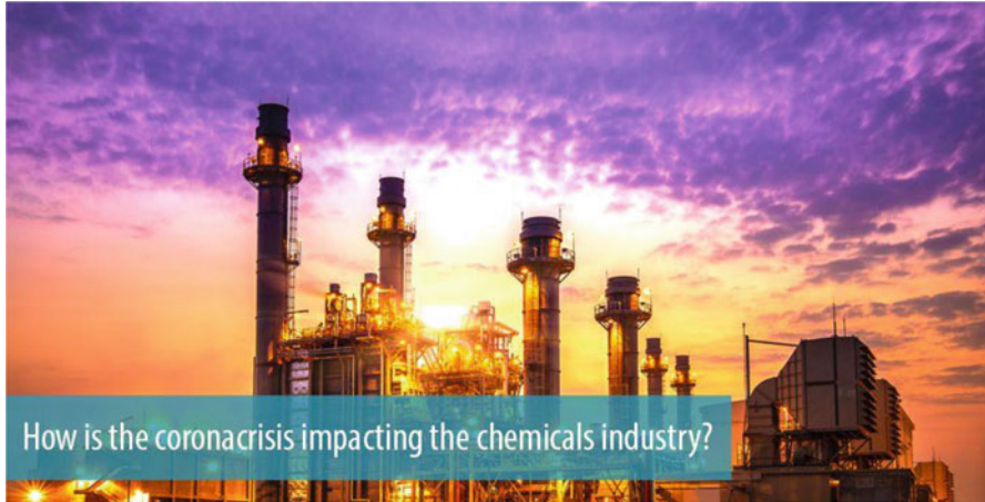
Fig. 11.4 Oil, gas, and chemical sector
