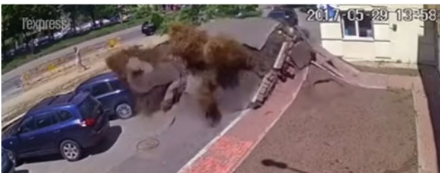
Fig. 2 Pipe burst in Kiev ( https://www.youtube.com/watch?v=Agb_pboPhBs )
