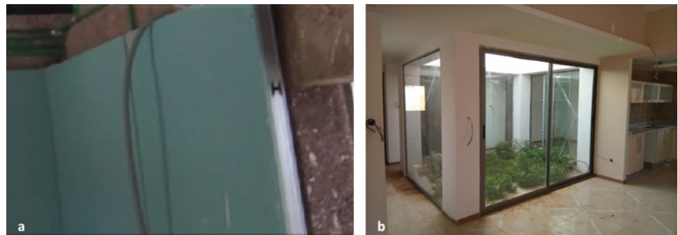
Fig. 4 Internal insulation of walls (a), Double-glazed window doors (b)
