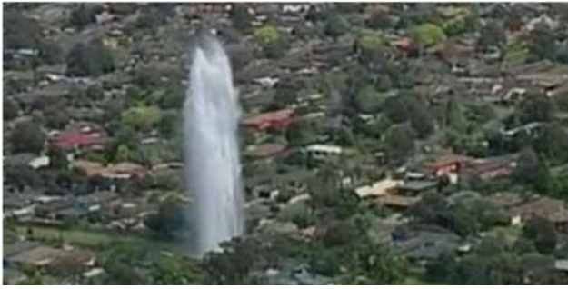
Fig. 1 Pipe burst in Melbourne ( https://www.planet.fr/international-video-lexplosion-spectaculaire-dune-conduite-deau-en-australie.262572.29335.html?page=0%2C1 )
