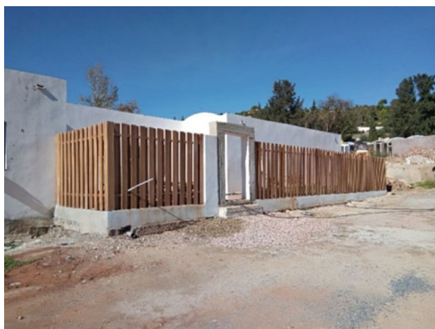
Fig. 2 Experimental bungalow, Hammam Righa spa, Algeria
