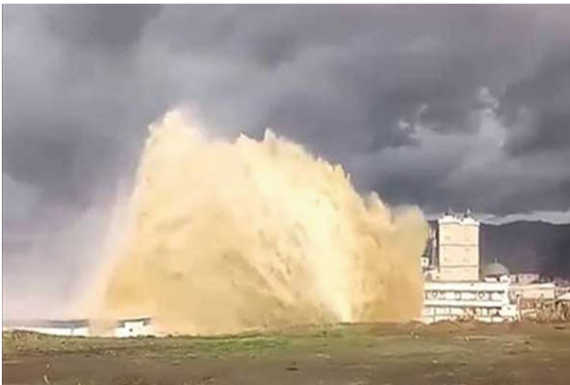
Fig. 3 Pipe burst in Djebahia ( https://www.express-dz.com/2018/11/27/bouira-explosion-spectaculaire-dune-conduite-deau-a-la-station-de-pompage-de-djebahia/ )
