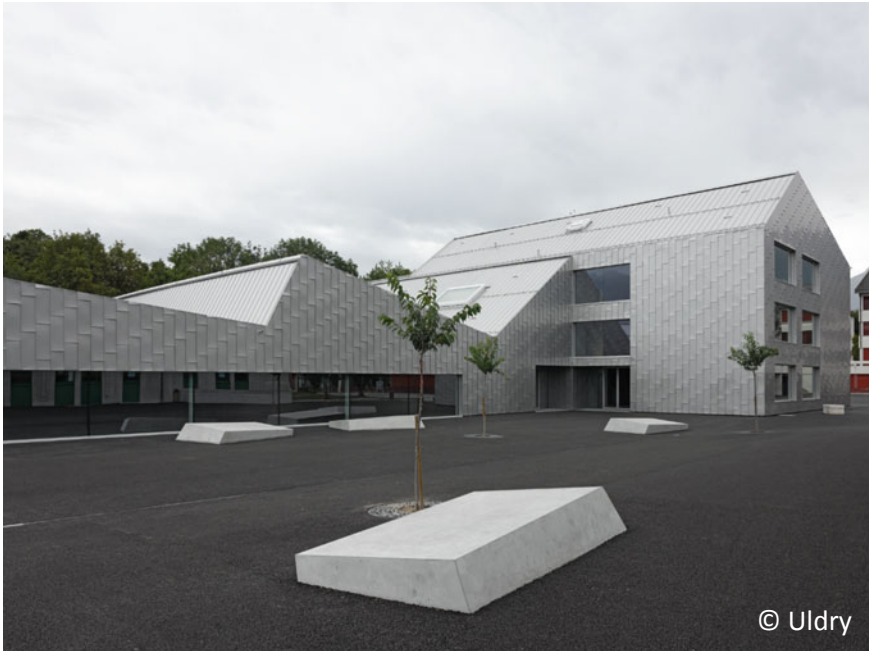
Fig. 12.1 The considered school-demo building, composed by two joint volumes. On the left part of the picture, it can be seen the gym volume, while, on the right side, there are the classrooms. The pure line of the building is part of the architectural language defined to draw the building at the macro scale, to guarantee the wished “monolithic” form and a dialogue with the surrounding alpine environment and traditional village shapes
