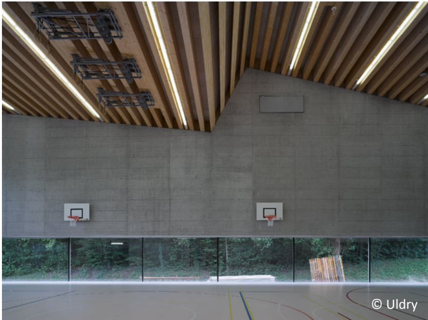
Fig. 12.3 The assumed design solution, able to respect architect's requirements for pure glazed openings, was to dissociate air paths from light paths. The picture shows an opaque opening on the top of the space, which guarantees the evacuation of hot air from the top and avoid the creation of a hot buffer space under the roof triangles. Glazing systems on the bottom offer only light and view, without being included in the natural ventilation solution
