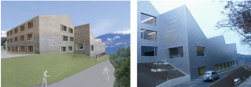
Fig. 12.4 On the left picture, it is possible to see the building as it was on the architectural contest poster. On the right as it was realised. The only difference is the opaque windows that can be only be guessed—see for example the top of each triangular roof of the gym and the vertical façade on the right picture
