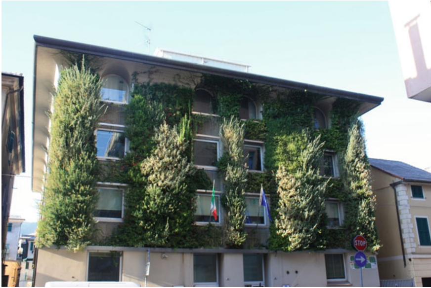
Fig. 10.4 The pilot project INPS Green Façade, Genoa (Italy)
