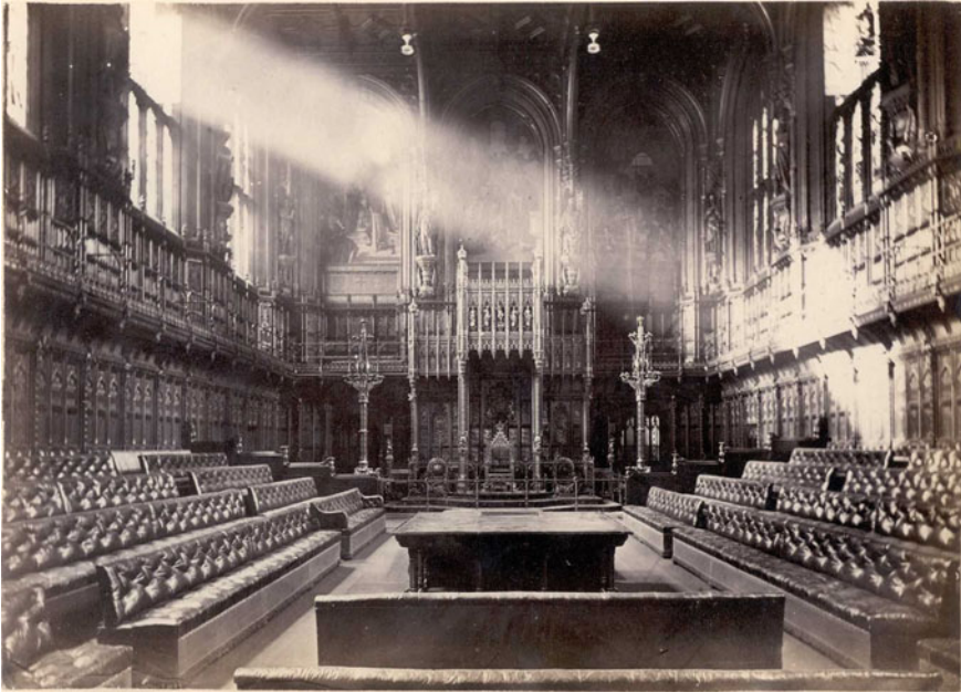
Fig. 13.11 Historic photographs, 1868, showing the interior of House of Lords with open windows admitting sunlight (British Library)
