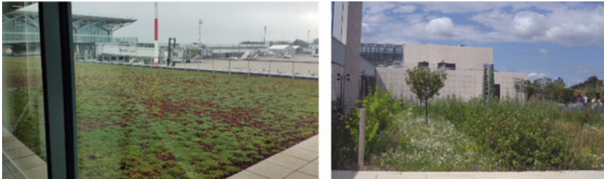
Fig. 10.1 Left: Extensive green roof. Zurich (Switzerland) 2017. Right: Intensive green roof. Greenwich (UK) 2015
