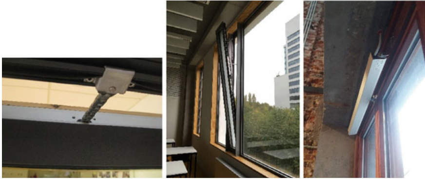
Fig. 6.2 Examples of chain actuators to open a window in Solstad Kindergarten in Norway (left) [25] and office buildings in Belgium (middle and right)
