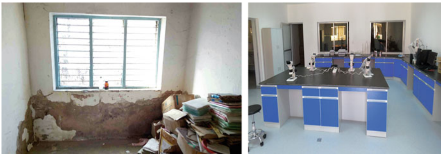
Fig. 14.9 Before and after the renovation of the laboratory
