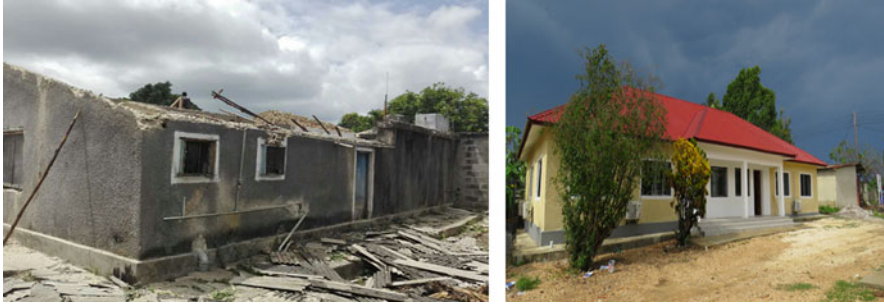
Fig. 14.8 Before and after the re-construction of the office building
