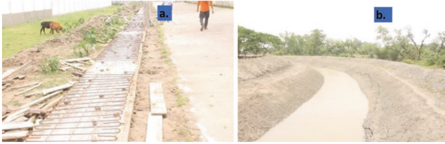
Fig. 2.15 Current structural and nonstructural measures. (a) Roadside drainage. (b) Excavation channel
