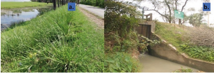
Fig. 2.16 Current resilience measures. (a) Planting vetiver grass. (b) Sluice gate for water regulation (Patuakhali)
