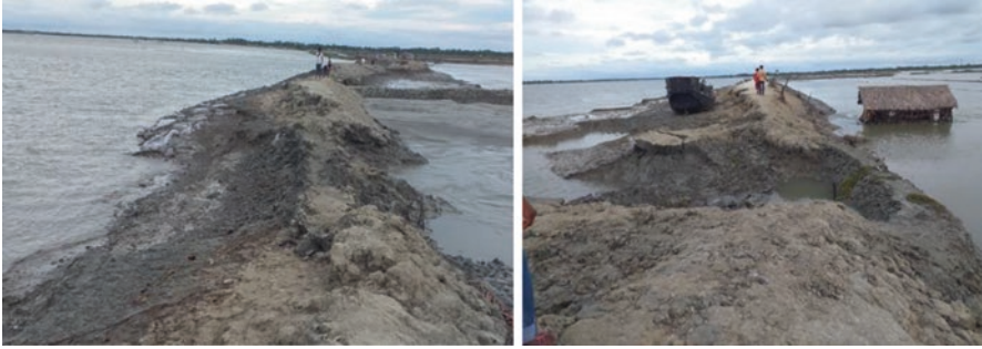
Fig. 2.11 Super cyclone “Amphan” washes out earthen embankment in Satkhira District (Field Survey: 10 June 2020)
