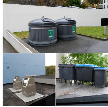
Fig. 2. Types of waste bins (top-Standard underground waste bins, left bottom-Sensor-based underground bins, right bottom-normal bins)
