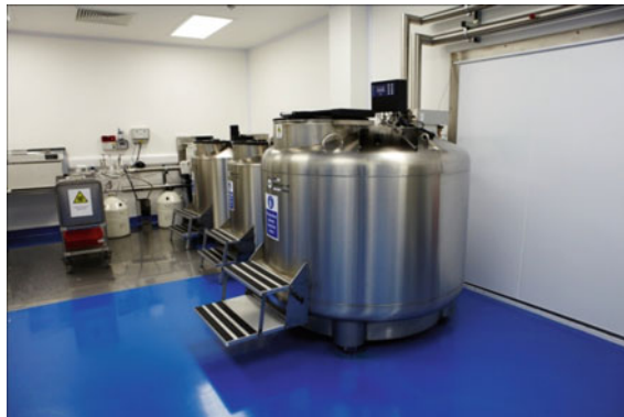
Cryogenics area in Anthony Nolan cell therapy centre-UK (Picture taken by Stephen Pennells)
