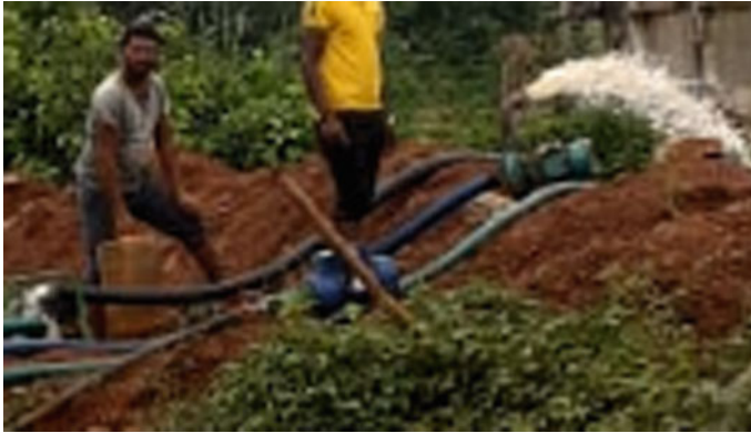
Fig. 20.16 Worker doing water supply work
