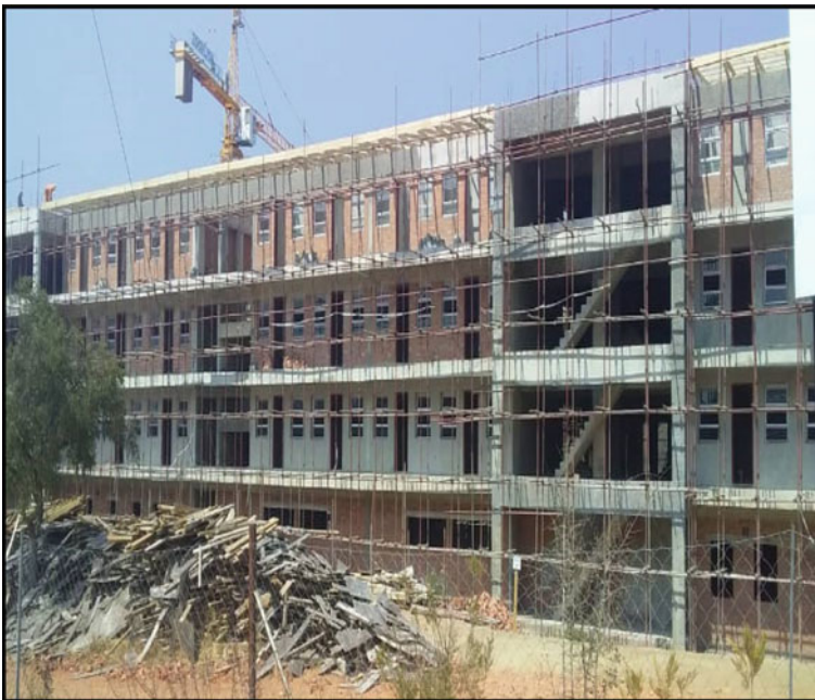
Fig. 4.3 Student hostel being constructed by the Infrastructure Development Bank of Zimbabwe
