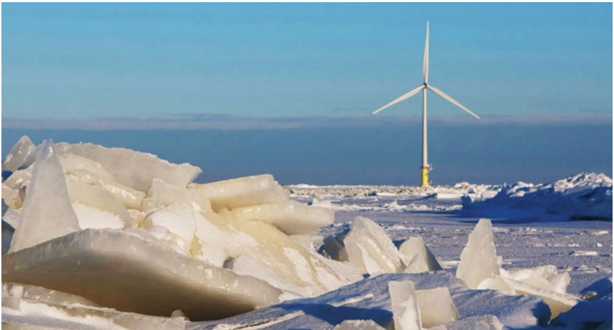
Fig. 10.2 An ice-resistant steel wind turbine foundation with gravel infill in icy waters in the Gulf of Bothnia (Hyötytuuli 2020)
