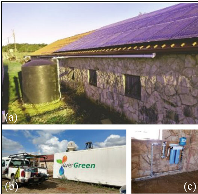
Fig. 6 (a) Rain gutter and 3000-gallon main reservoir, (b) vertical farming unit, and (c) filtration unit
