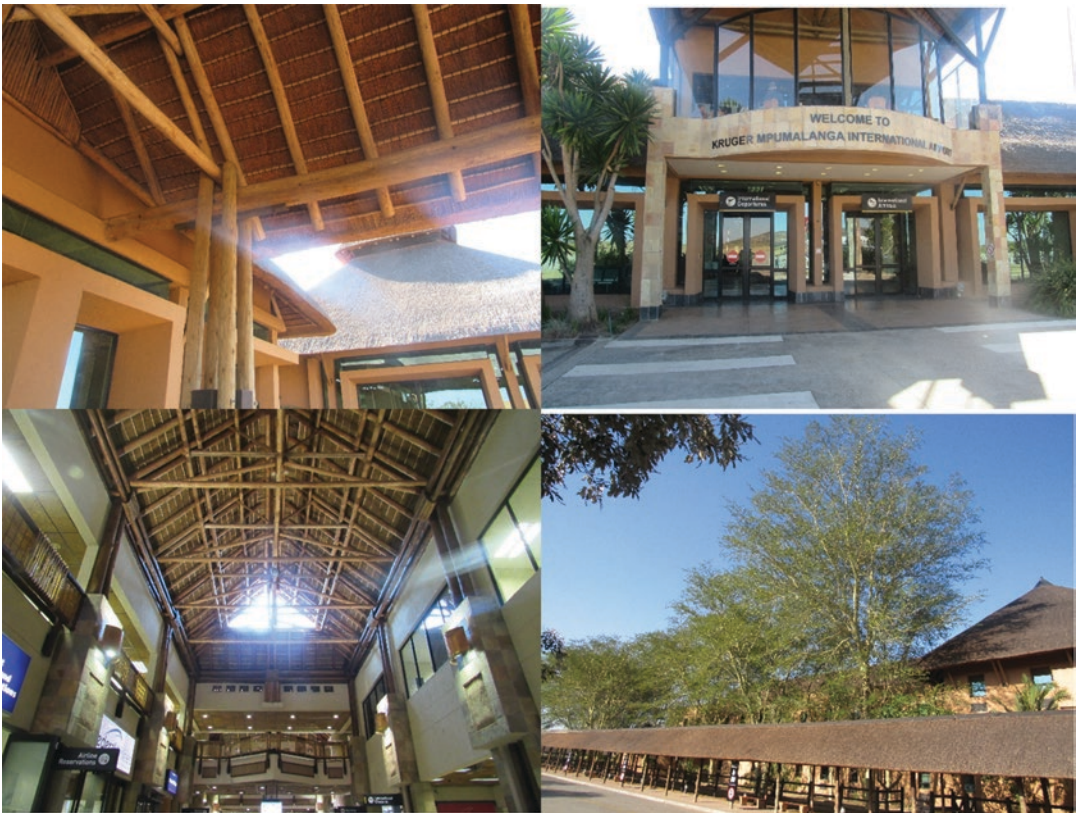
Fig. 12.4 Kruger Mpumalanga is one of the few thatched roof airports in the world. (Source: Based on fieldwork (2019))
