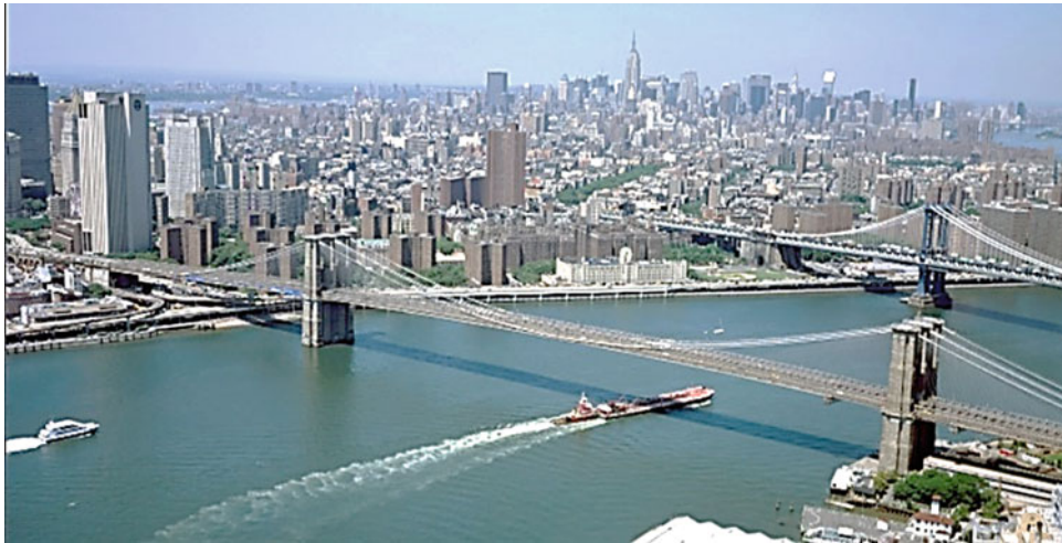
Fig. 19.11 Photograph of typical suspension bridge normally WAS with zinc coat followed by painting for environmental protection against corrosion
