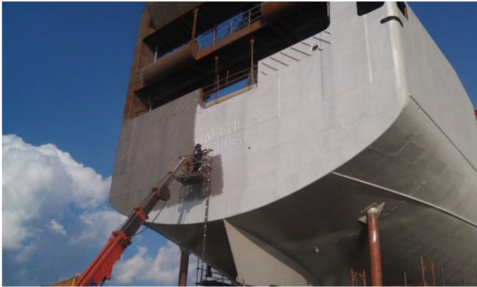
Fig. 11.60 Zinc arc spraying of Norwegian fishing trawler using Arcspray 140 system. http://www.metallisation.com/
