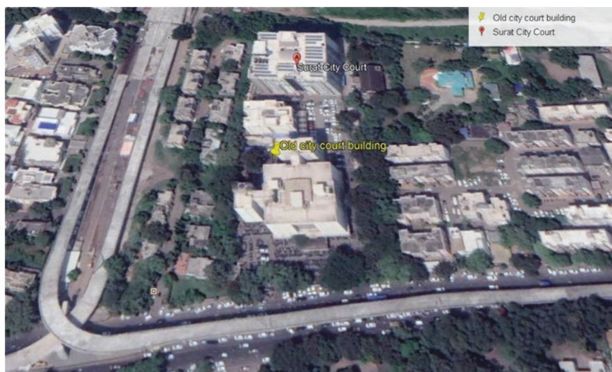
Fig. 1. Demolition site of District (City) Court.
