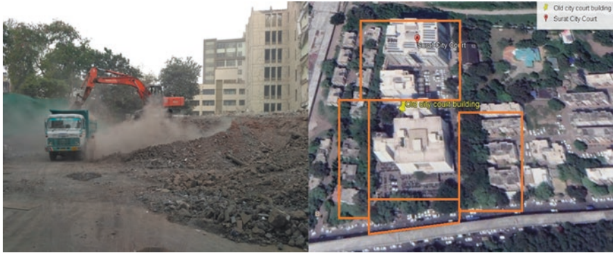
Fig. 4. Neighbourhood nuisance due to demolition activities.
