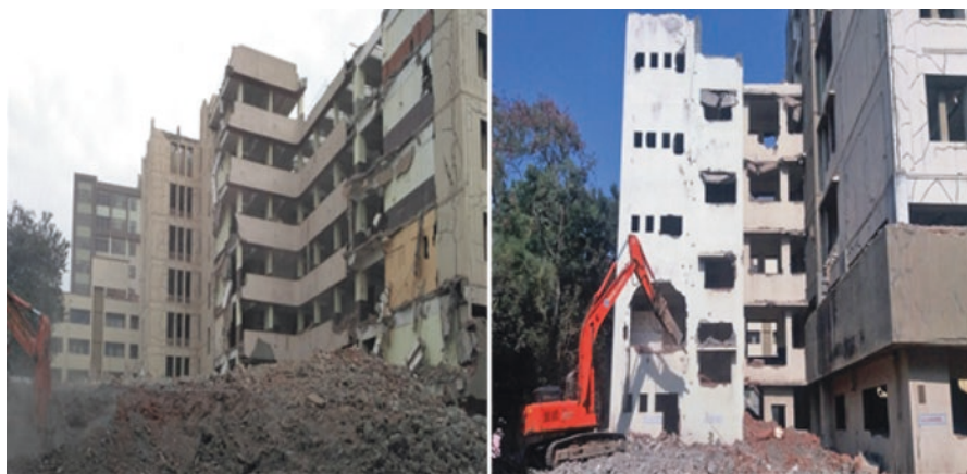
Fig. 3. Semi-mechanised demolition operations.
