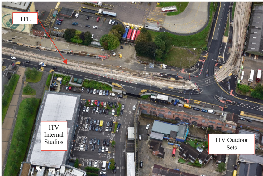
Fig. 1. Aerial view of site
