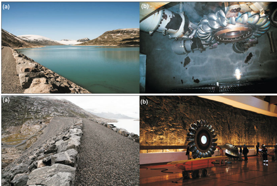
Fig. 10.7 Top a Styggevatn reservoir in upper Jostedal in western Norway. Although an exception with a glacier Austdalsbreen (still) calving into the reservoir, many reservoirs in Norway have inflow from glaciated catchments at variable percentages. b Pelton wheel and water nozzles of the Jostedal hydropower plant build deep into the bedrock of the valley side. The water utilised
