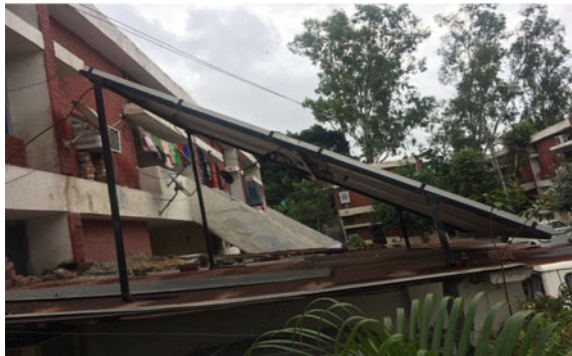
Fig. 5 Solar panels mounted at optimum angle
