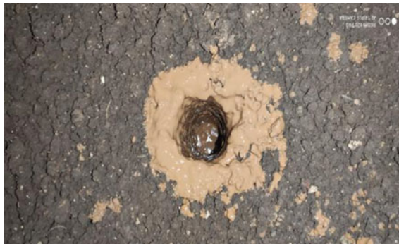
Fig. 3 Application of Bentonite Slurry
