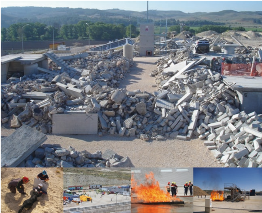
Fig. 26.3 Practice area for first responders in Madrid area, where the technologies of FASTER will be evaluated during the Spanish pilot
