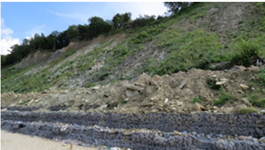
Fig. 2. 2012 Destruction of the lower stage after a storm.
