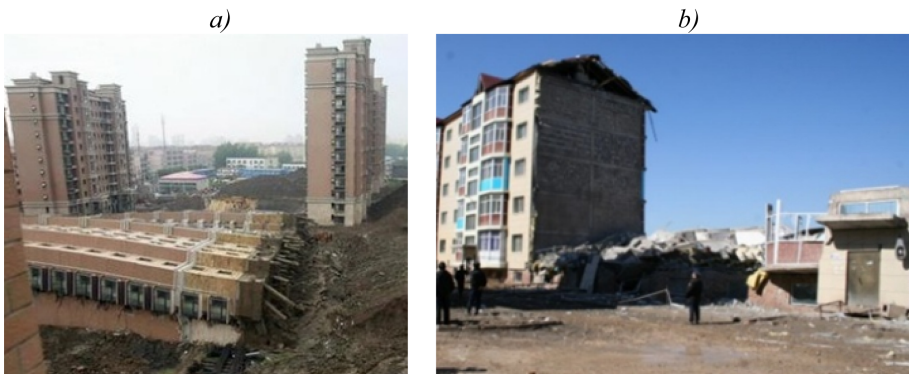
Fig. 1. Examples of building collapses due to loss of stability; (a) the fall of a multistoried building in China (Shanghai 06.2009); (b) collapse of a new building in Karaganda (04.2012).
