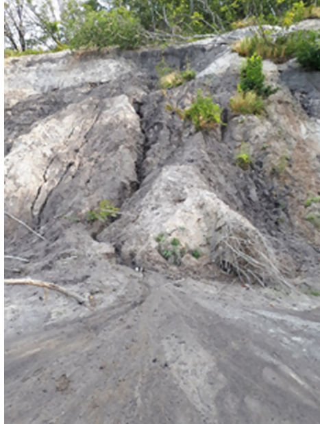
Fig. 5. 2019. The soils composing the slope, in areas not fixed by gabions, have undergone partial slumping and suffusion.
