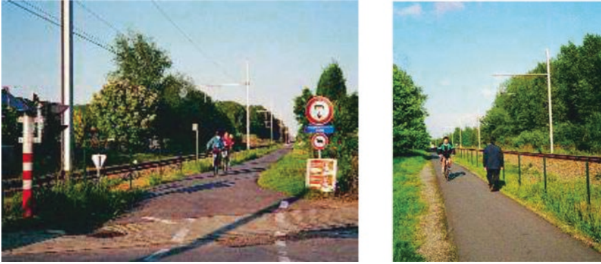
Fig. 3 The Puurs Greenway represents a good example of coexistence between an active railway line and a greenway. Source: European Greenways Association (1998)
