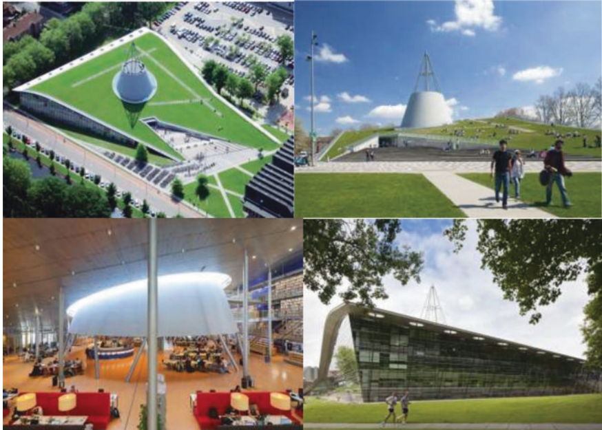
Fig. 13 The library is a building that does not really want to be a building, but a landscape (Mecanoo 2019)
