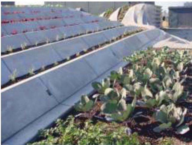
Fig. 10 Architectural integration of the green roof with edible plants, example of the complex roofs
