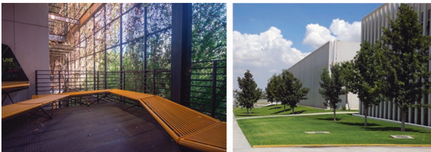
Fig. 12 Vegetable cover on a green wall shading a resting place (left) and a grass cover in a garden surrounding a building (right) (source: own work)
