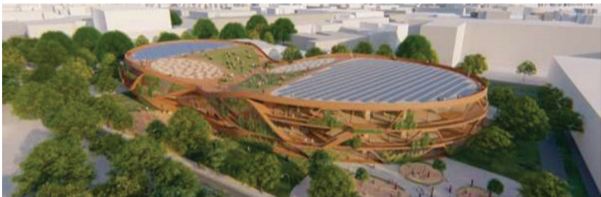
Fig. 23 External view of the building with the photovoltaic plants and the edible food garden
