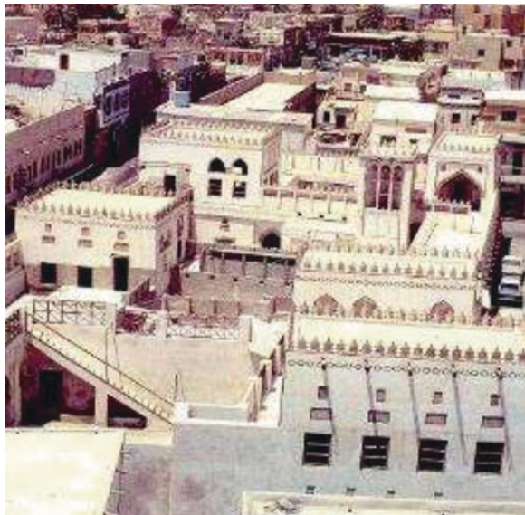
Fig. 2 Compact buildings in a traditional town increase the shade and wind movement on roads
