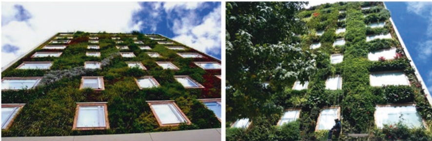
Fig. 36 Vertical gardens (green walls) of Hotel B3, Bogotá, Colombia. (Image source: https://tropicalcommons.co/en/2018/09/04/vertical-gardens-and-green-roofs-of-colombia/ )
