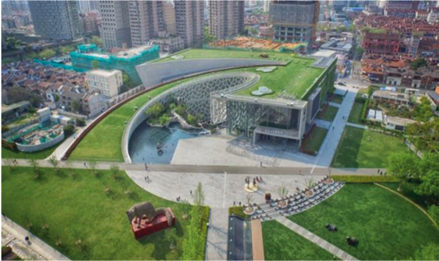
Fig. 42 Green roofs Shanghai's Natural History Museum. (Images source: https://cdn.archpaper.com/wp-content/uploads/2015/04/01_Shanghai-Natural-History-Museum.jpg )
