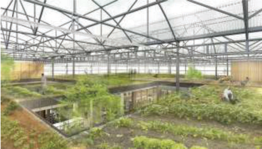
Fig. 22 The integrated rooftop greenhouse (IRTG), resulting after connecting a rooftop greenhouse to the underneath building, by controlled flows of energy, water, and gases: O 2 -enriched air from rooftop greenhouse to building and CO 2 -enriched air from building to the rooftop greenhouse. IRTG supports an efficient integrated management of energy, water, CO 2 , and O 2 that collects the disposable renewable energy resources: sun (by greenhouse effect), wind (by air-to-air heat pumps), geothermal (by water-to-water air heat pumps), and water resources (rainwater, household grey water, water vapours), storing and delivering them wherever and whenever needed inside the IRTG system
