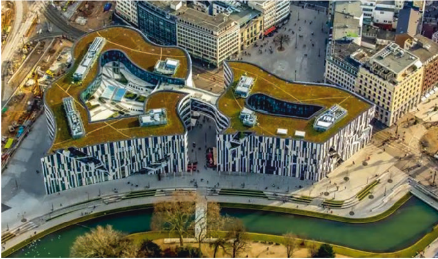
Fig. 12 Green roofs of Kö-Bogen retail and office complex, Düsseldorf, Germany. (Image source: https://www.theguardian.com/cities/gallery/2018/aug/17/urban-oases-green-roofs-around-the-world-in-pictures )
