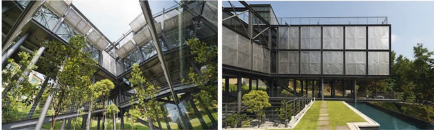
Fig. 73 Green roof of Cantilever House, Malaysia. (Images source: https://inhabitat.com/green-roofed-cantilever-house-floats-above-the-malaysian-rainforest/cantilever-house-by-design-unit-sdn-bhd-3/ )
