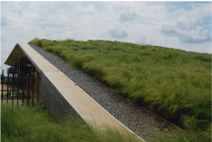
Fig. 89 Green roof at DBSA, South Africa. (Image source: https://i.pinimg.com/originals/ee/f7/06/ee706f0df50be6e33ae7acfcc29b122.jpg )
