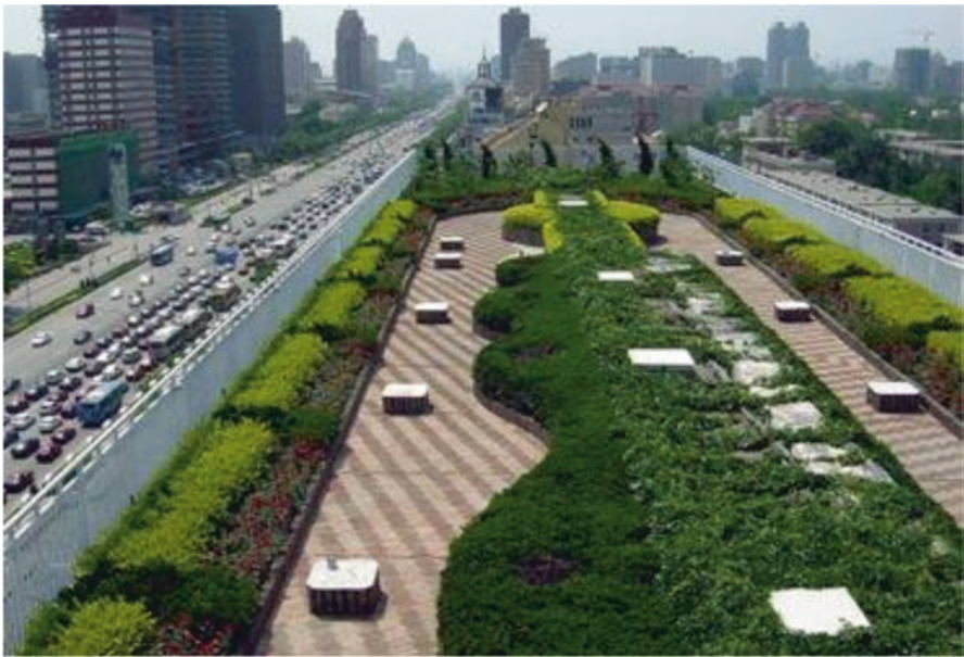
Fig. 45 Green roofs of Beijing's Chemical Mansion and Sunshine Mansion, China. (Images source: https://www.treehugger.com/corporate-responsibility/chinas-learning-to-love-green-roofs.html )
