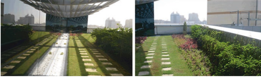
Fig. 94 Rooftop green roof of Dubai Silicon Oasis Authority’s building, UAE. (Images source: http://www.hillsandfort.com/landscape/gallery.php?portId=15&page=projects )
