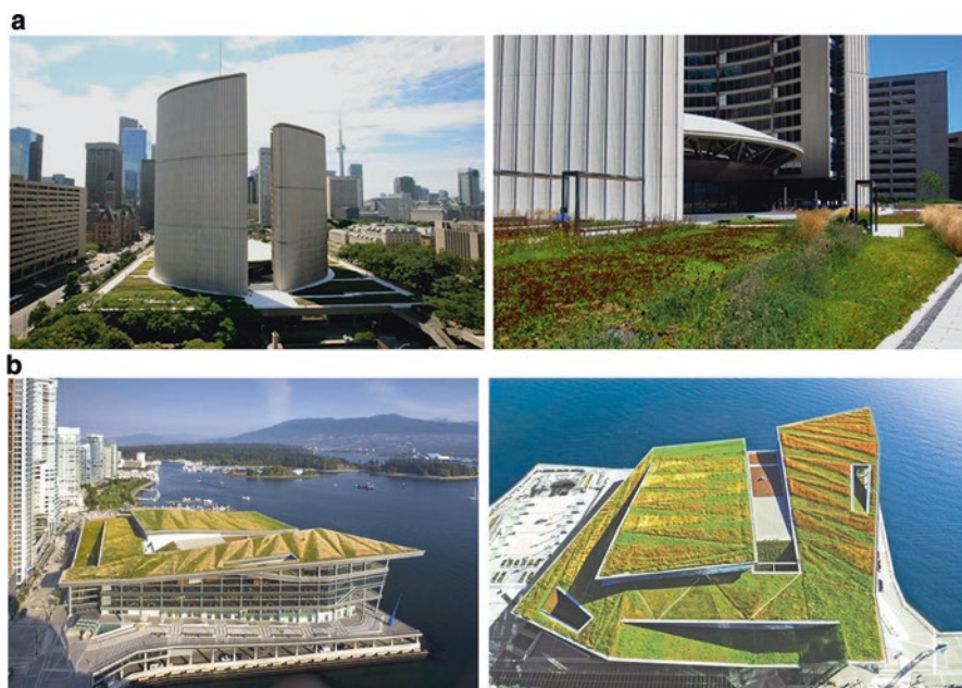
Fig. 30 Green roofs in Toronto and Vancouver, Canada. (a) Green roofs of City Hall podium in Toronto. (b) The Convention Centre green roof—waterfront at Canada Place in Vancouver. (Images source: https://www.greenroofs.com/projects/nathan-phillips-square-toronto-city-hall-podium-green-roof/ ; https://www.skyluxe-roofing.com/green-flat-roof/ ; https://www.goodnet.org/articles/5-impressive-green-roofs-from-across-globe . https://torontoimages.wordpress.com/2011/07/15/green-roof-toronto-city-hall/ )
