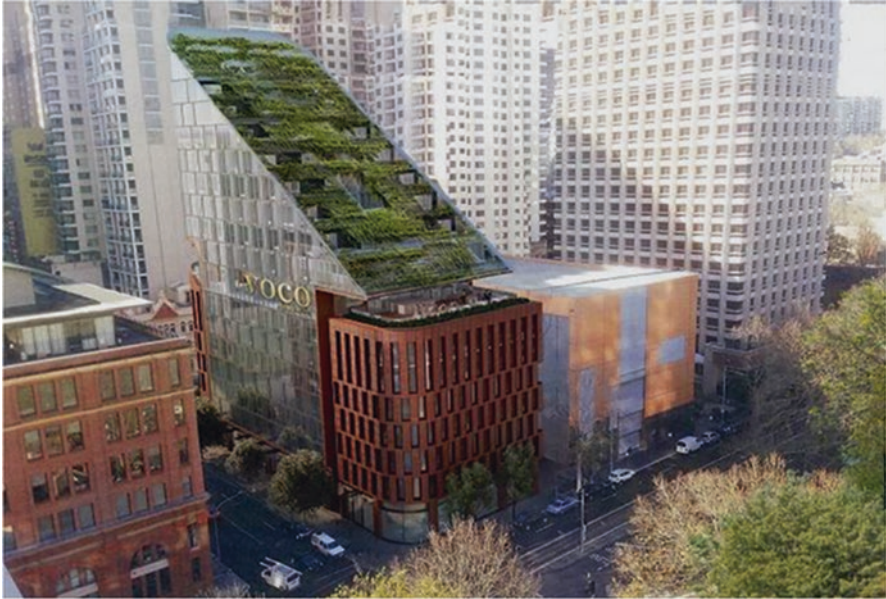
Fig. 78 Green roof of the new VOCO hotel in Sydney, Australia. (Images source: https://www.traveltalkmag.com.au/hotels-and-resorts/sydneys-newest-hotel-boasts-outdoor-green-waterfalls )
