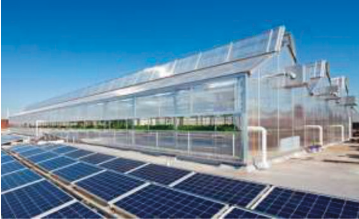
Fig. 16 View of the rooftop greenhouse with the photovoltaic plant. The electrical needs of Gotham’s current Greenpoint greenhouse facility are met, in part, by a 56 kW on-site solar PV system that produces 70,000 kWh of electricity annually
