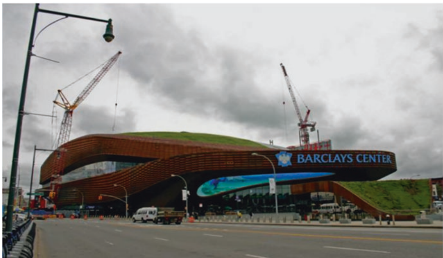
Fig. 28 Barclays Center's green roof, Brooklyn, Lower Manhattan—New York, USA. (Image source: https://archpaper.com/2015/06/gallery-barclays-centers-green-roof-sedum-installation-50-complete/ )
