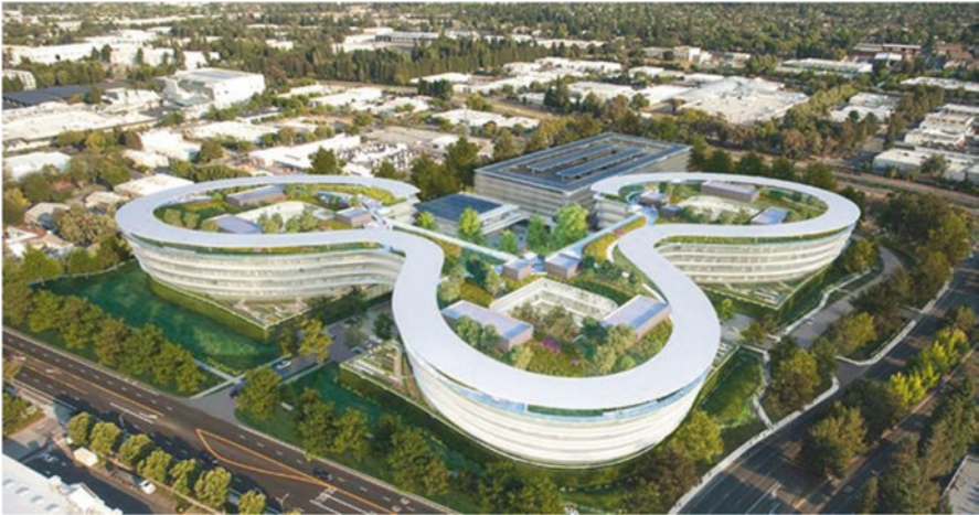
Fig. 24 Large green roofs on Apple new office building in Silicon Valley, California, USA. (Image source: https://www.dezeen.com/2015/10/07/apple-silicon-valley-campus-hok-california-green-roof/ )
