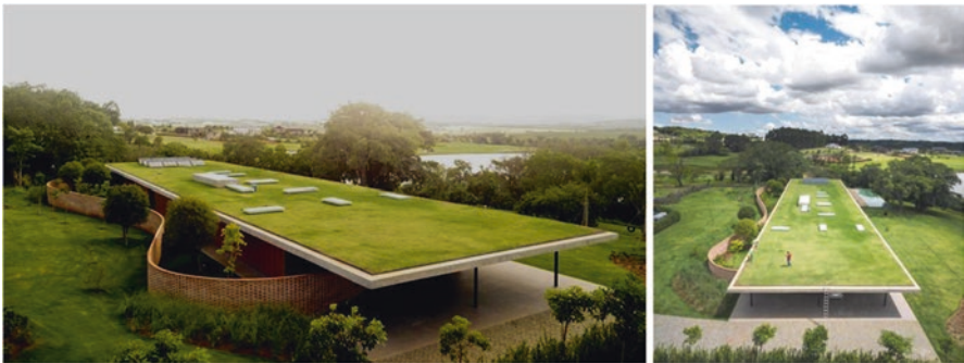
Fig. 32 Green roofs of Studio MK27 outside São Paulo, Brazil. (Images source: https://worldarchitecture.org/architecture-news/ehfvq/studio-mk27-completes-planar-house-with-extended-green-roof-outside-of-so-paulo.html )
