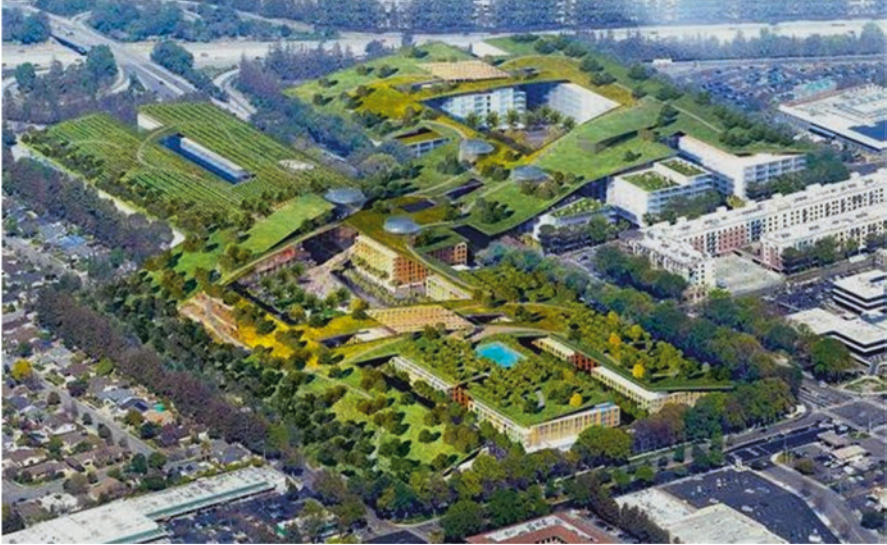
Fig. 23 The largest rooftop garden in Silicon Valley, San Francisco—California, USA. (Image source: https://www.pinterest.co.uk/pin/66639269464234105/ )
