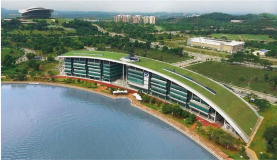
Fig. 75 Green roof of Heriot-Watt University campus in Putrajaya, Malaysia. (Images source: https://www.hw.ac.uk/about/work/malaysia.htm )
