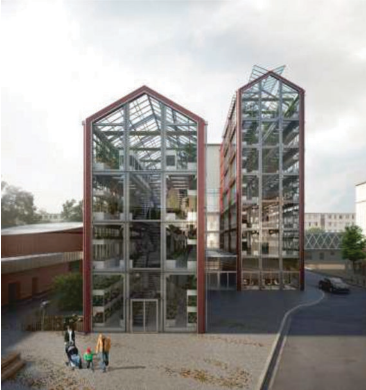
Fig. 44 General view of the building (photo Ilimelgo )
