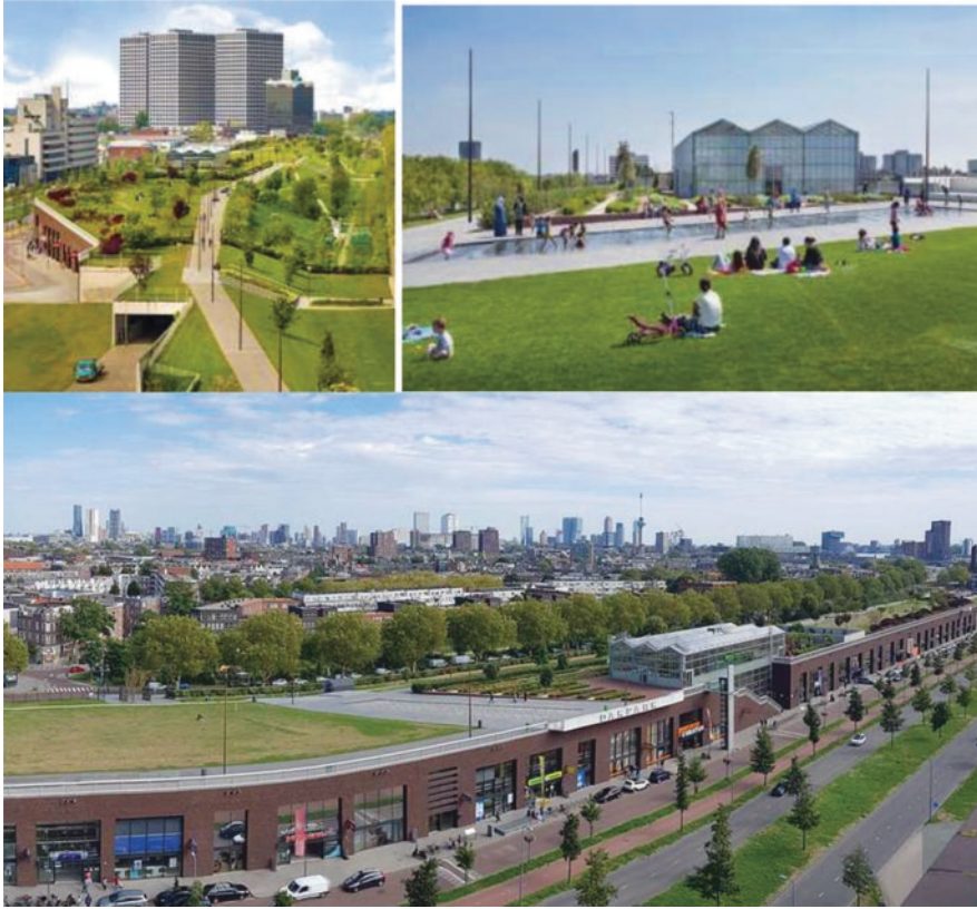
Fig. 16 Roof park Vierhavenstrip—Rotterdam
