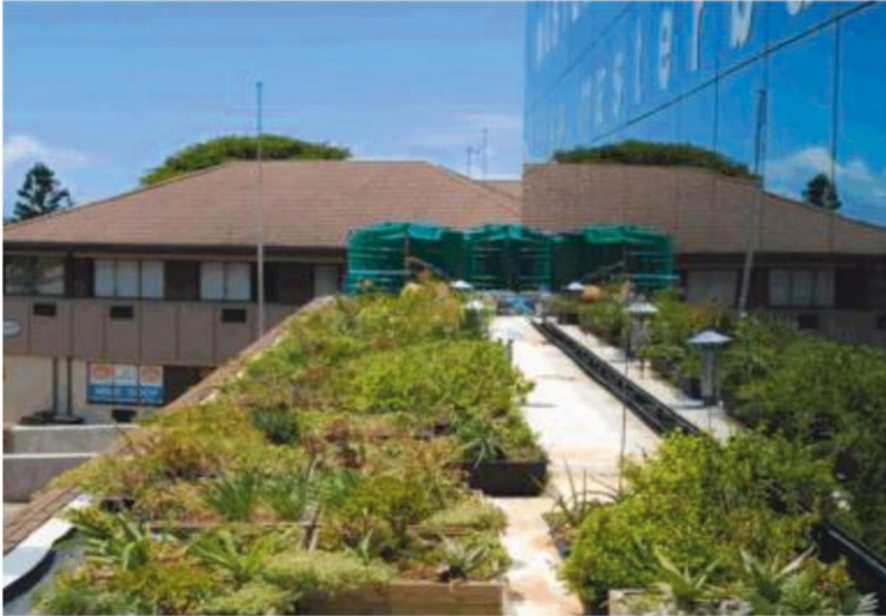
Fig. 90 Green roof of Master Builders Centre in Durban, South Africa. (Image source: https://www.greenroofs.com/projects/master-builders-association-durban-westville/ )
