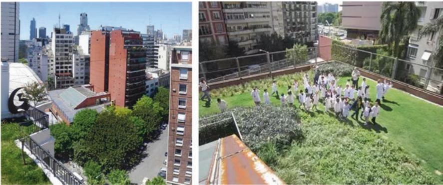
Fig. 34 Green roofs in Buenos Aires, Argentina. (Images source: https://www.lafargeholcim-foundation.org/projects/green-roofs-buenos-aires-argentina )
