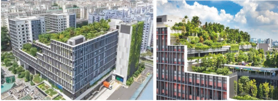
Fig. 71 Rooftop garden and green roof of an integrated mixed-used development—Kampung Admiralty’ in Singapore. (Images source: https://www.designboom.com/architecture/woha-kampung-admiralty-singapore-10-30-2018/ )
