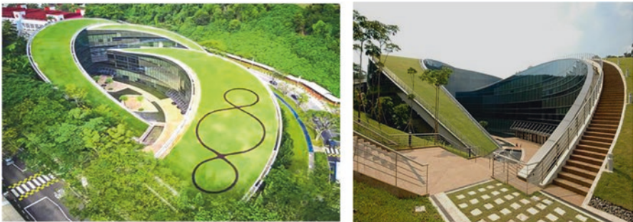
Fig. 70 Green roof of the School of Art, Design and Media (ADM) at Nanyang Technological University in Singapore. (Images source: http://news.ntu.edu.sg/pages/newsdetail.aspx?URL=http://news.ntu.edu.sg/news/Pages/NR2019_Jan_21.aspx&Guid=96eb2d18-367e-4f08-a96f-6053da41c852&Category=News+Releases )
