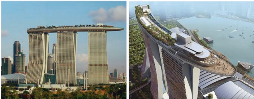
Fig. 67 Green roof of Marina Bay Sands, in Marina waterfront bay in Singapore. (Images source: https://www.greenroofs.com/projects/marina-bay-sands-integrated-resort-skypark/ ; https://mcf-consultoria.com.br/blog/?p=658 )
