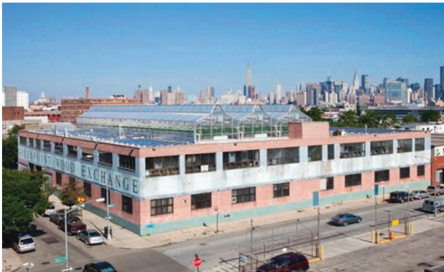
Fig. 17 General view of the building with greenhouses and the PV plant
