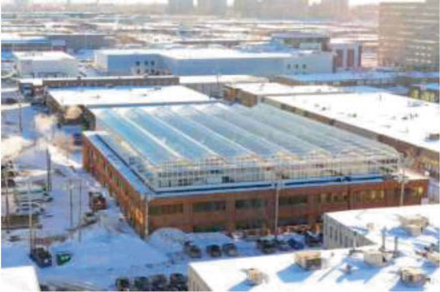
Fig. 34 General view of the building with the roof greenhouses in Montreal
