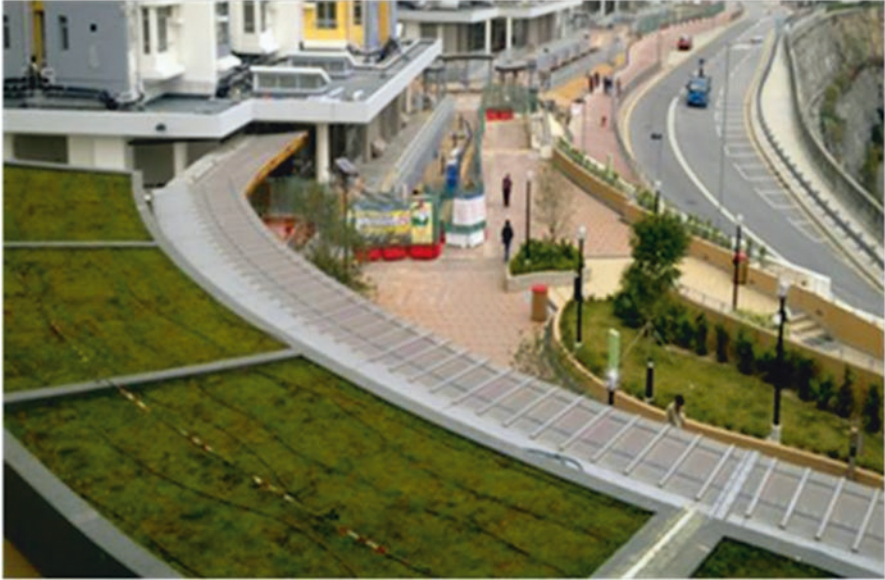
Fig. 54 Green roofs of residential buildings in Hong Kong, China. (Images source: https://www.sempergreen.com/us/references/housing-authority )
