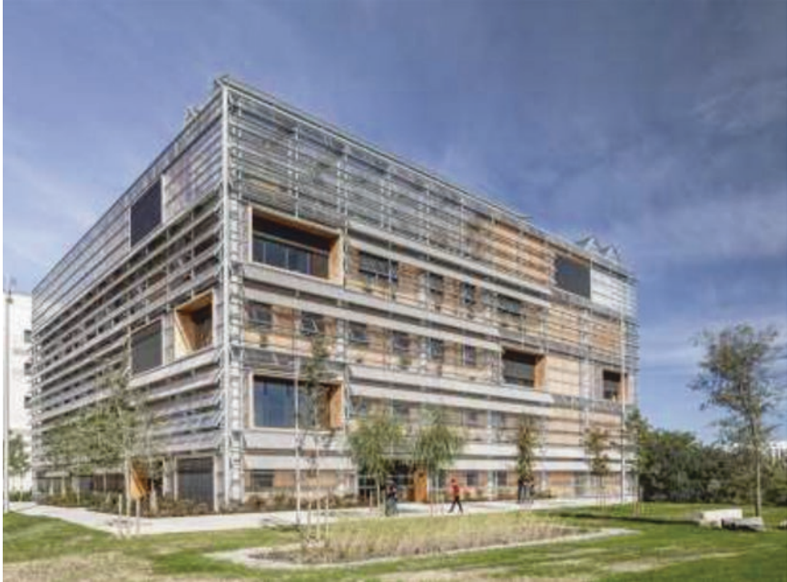
Fig. 31 ICTA-ICP building, general view
