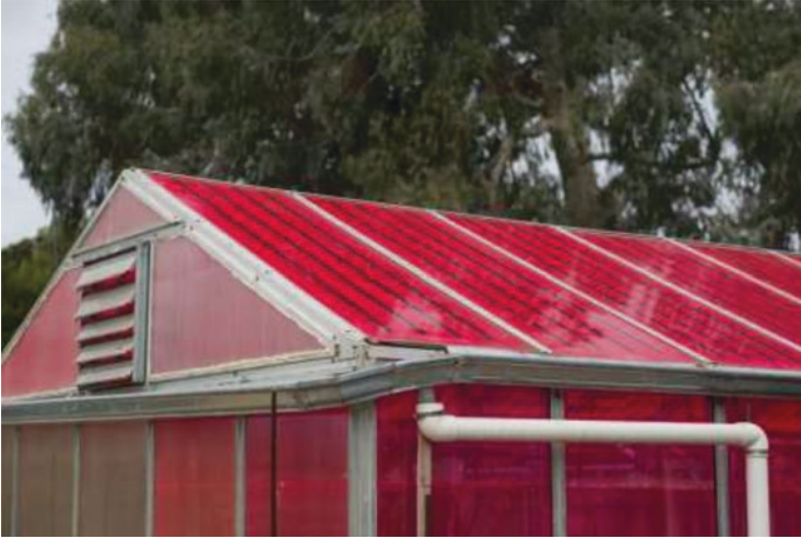
Fig. 2 Greenhouse integrated with solar energy panels; red modules help plants to optimize photosynthesis
