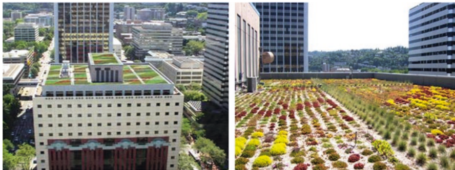
Fig. 19 City Building's green roof in Portland—Oregon, USA. (Images source: https://www.greenroofs.com/projects/the-portland-building/ )
