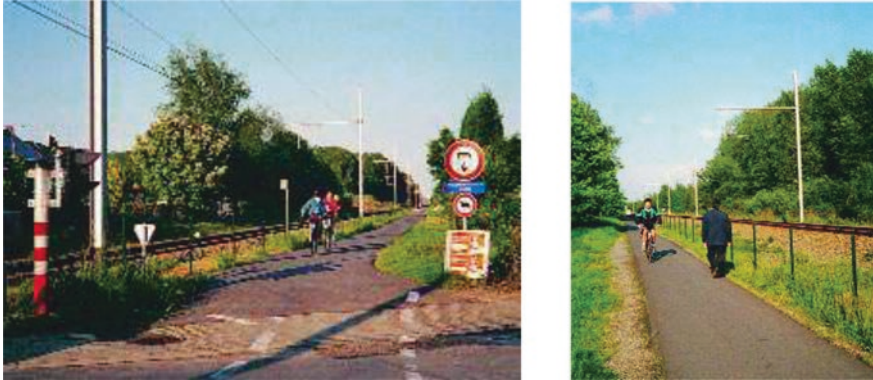
Fig. 3 The Puurs Greenway represents a good example of coexistence between an active railway line and a greenway. Source: European Greenways Association (1998)
