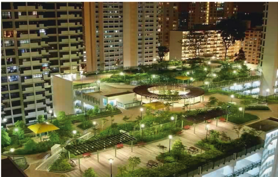
Fig. 72 Rooftop garden of block 38 in Jurong East, Singapore. (Images source: http://www.asiagreenbuildings.com/wp-content/uploads/2014/11/DAS9f5yCxmezqq1jmYCoF3NOo1_1280.jpg )
