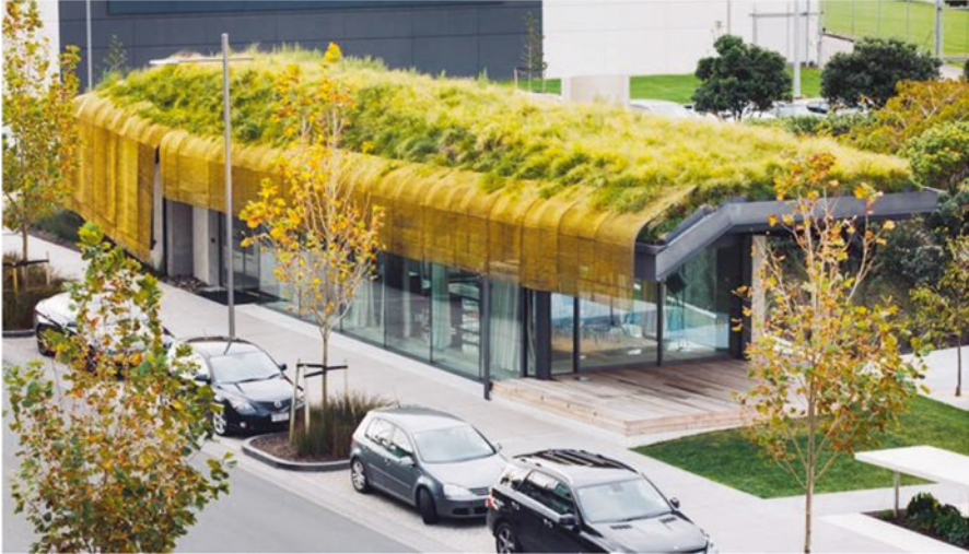
Fig. 86 Innovative green roof at Auckland International Airport, Auckland, New Zealand. (Image source: https://inhabitat.com/the-cloak-fearon-hay-architects-install-a-maori-inspired-green-roof-at-auckland-international-airport/te-kaitaka-the-cloak-fearon-hay-architects-2/ )
