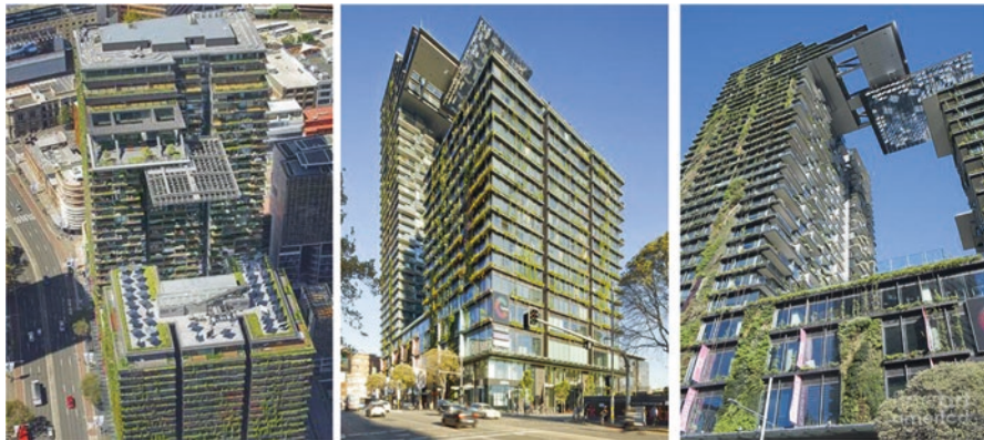
Fig. 77 Vertical gardens of One Central Park, Chippendale, a greenery high-rise building in Sydney, Australia. (Images source: https://urbannext.net/one-central-park/ ; https://fineartamerica.com/featured/one-central-park-chippendale-sydney-martin-berry.html )
