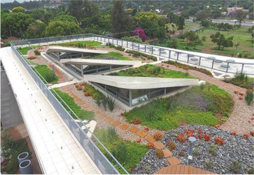
Fig. 88 Green roof at SANRAL, South Africa. (Images source: https://i.pinimg.com/originals/f3/11/eb/f311eb5fe90e237081cf62a38733358e.jpg )
