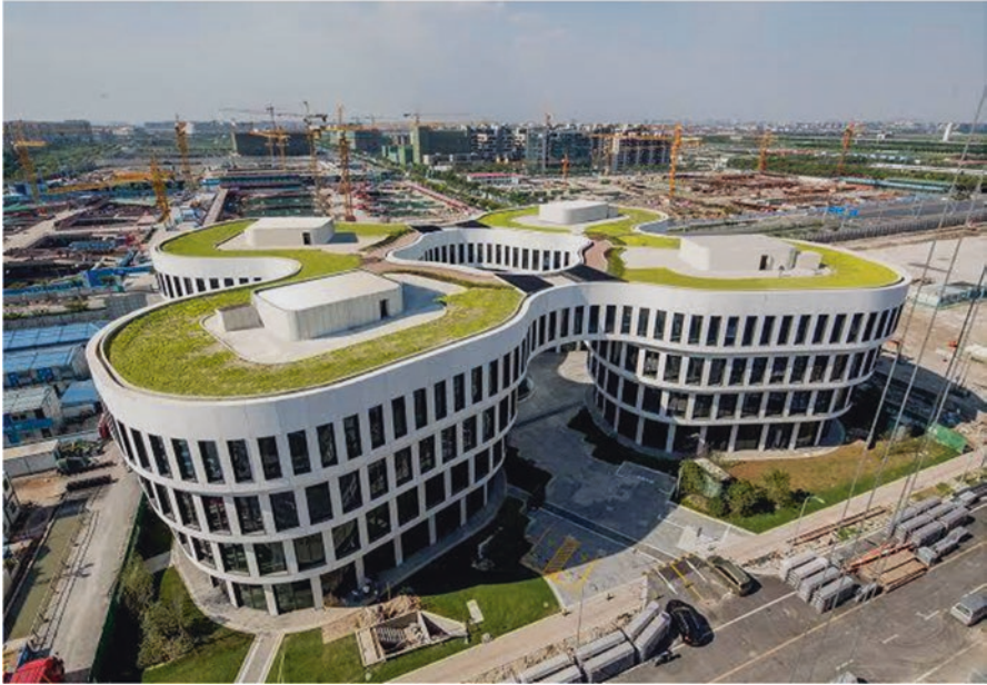
Fig. 44 Green roofs of Hongqiao Flower Building in Shanghai, China. (Images source: https://www.mvrdr.nl/projects/234/hongqiao-flower-building )
