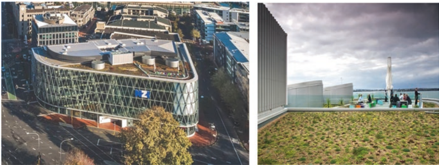
Fig. 85 Green roof of NZI Centre in Auckland, New Zealand. (Images source: https://www.colliers.co.nz/news/2018/green%20roofs%20could%20bring%20hidden%20costs/ )
