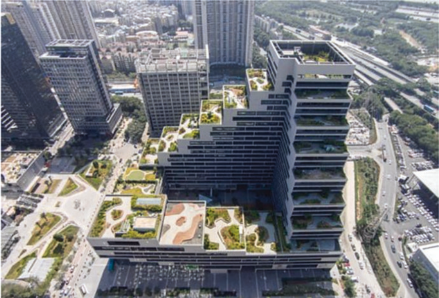
Fig. 51 Cascading green roofs in Shenzhen, China. (Images source: https://www.archdaily.com/788409/shenye-tairan-building-zhubo-design )
