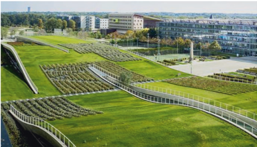
Fig. 16 École des Ponts ParisTech, school built under green roofs in Paris, France. (Images source: https://www.treehugger.com/green-architecture/green-roofs-are-changing-architecture-heres-whole-school-built-under-undulating-green-roof.html )
