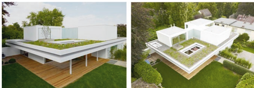
Fig. 8 Green roof of Studio S in Wiesbaden, Germany. (Source: (a) https://ar.smarthomemaking.com/20-green-walled-buildingsinspiring-your-own-plant-cladded-home . (b) https://inhabitat.com/3-rooms-3-trees-and-a-meadow-adorn-the-roof-of-house-s-in-germany/house-s-roger-christ-2/ )
