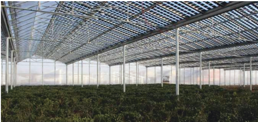
Fig. 1 Photovoltaic integration in a greenhouse for urban farming
