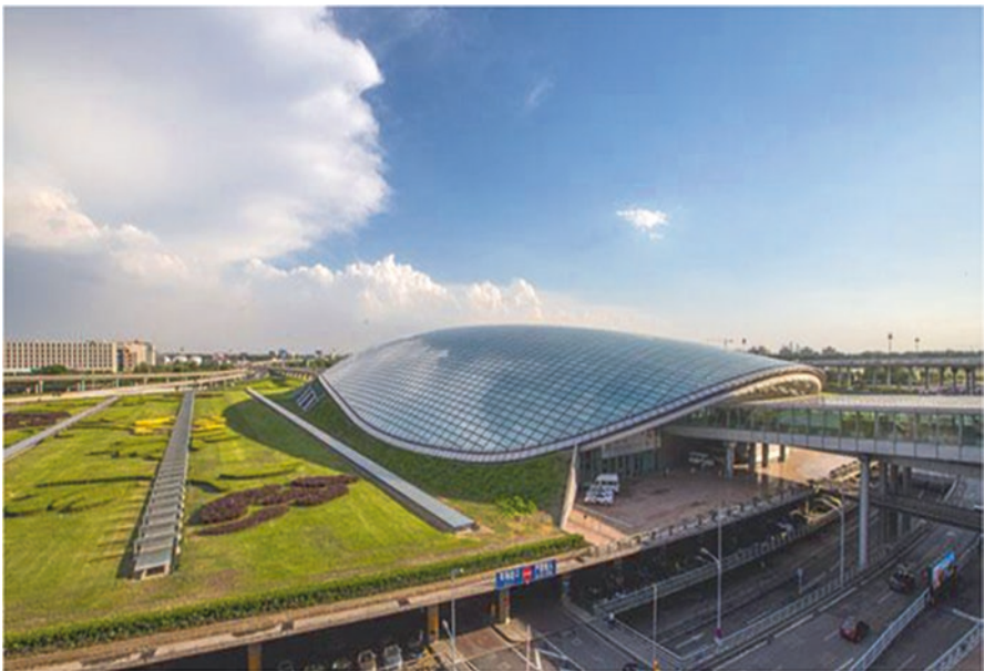
Fig. 49 Green roof of Beijing airport. (Images source: https://www.topchinatravel.com/beijing/how-to-spend-a-6-hour-layover-in-beijing.htm )
