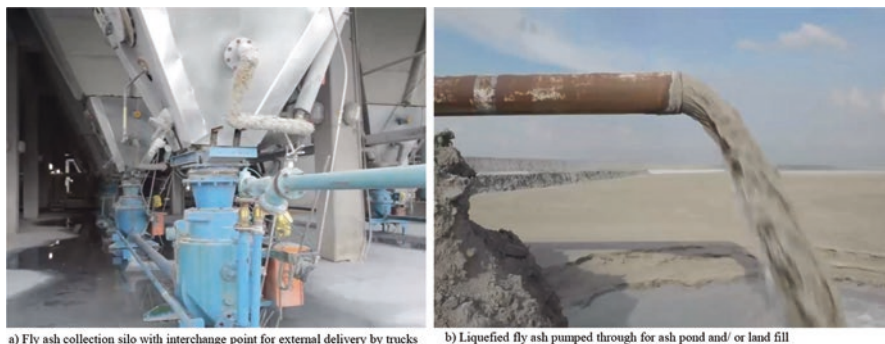
Fig. 15.3 Fly ash collection (a) and deposition (b)
