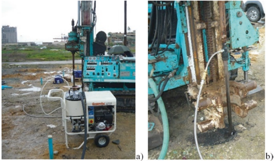
Fig. 13 (a, b) General aspect of the nZVI injection device
