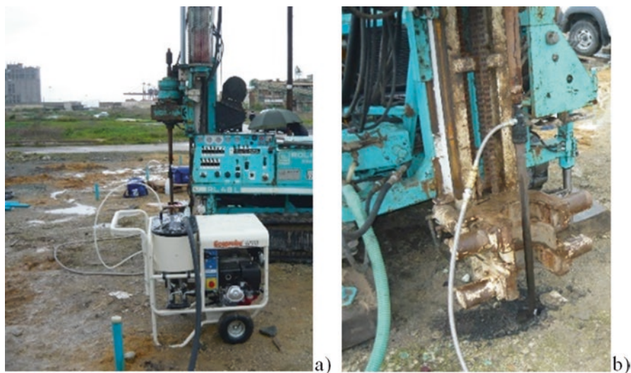
Fig. 13 (a, b) General aspect of the nZVI injection device
