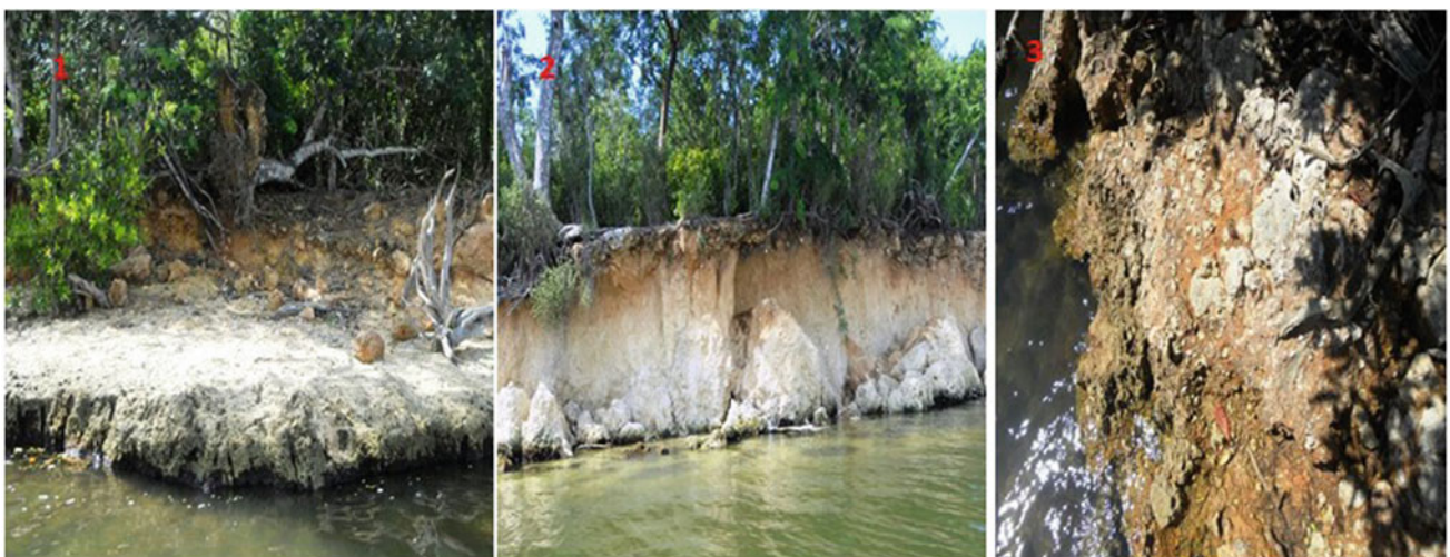
Fig. 2.17 Quaternary formations in Ocampo key, Cienfuegos bay. Jaimanitas Formation at the base of the cut covered by the La Cabaña Formation (from left to right, photos 1 and 2) and by the El Salado Formation (photo 3)
