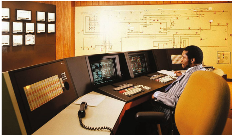
Fig. 1.4 Carolina Power and Light control room in the 1970s
