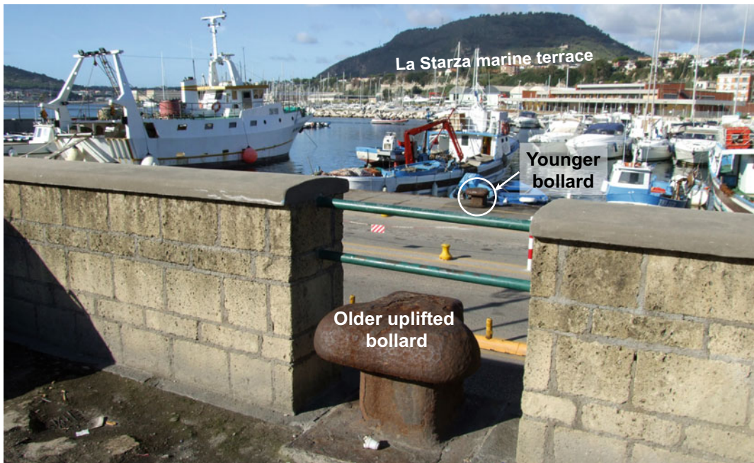
Fig. 5.15 Example of notable shorter- and longer-term deformation at Campi Flegrei caldera, Italy. Foreground: older dock level of the Pozzuoli harbour, in the caldera centre, uplifted of \sim 2 m during the 1982–1984 unrest, with the newer and currently active dock level, built after
