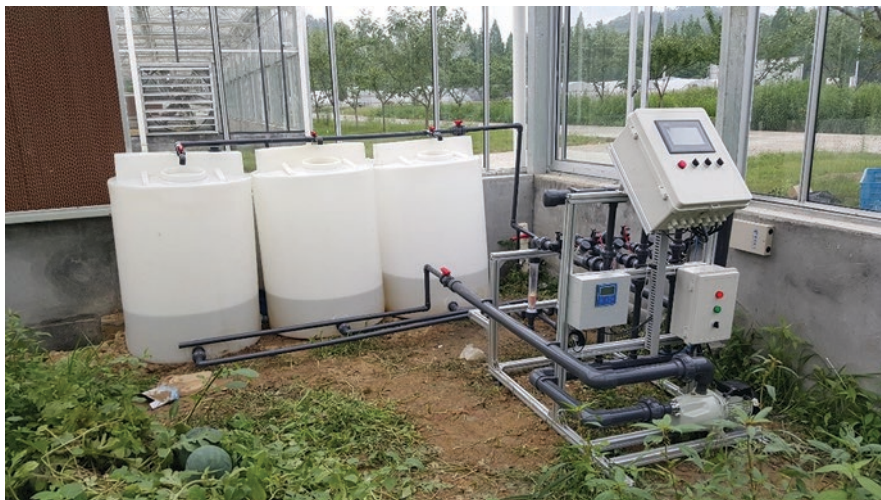
Fig. 11.11 Nutrient solution circulation and automatic control systems
