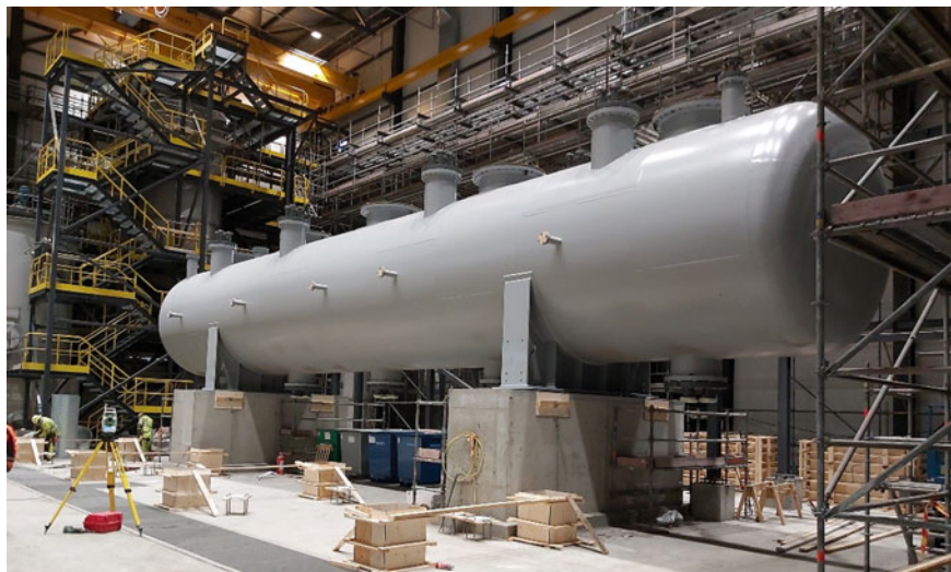
Fig. 3 The POX autoclave during installation. (Color figure online)
