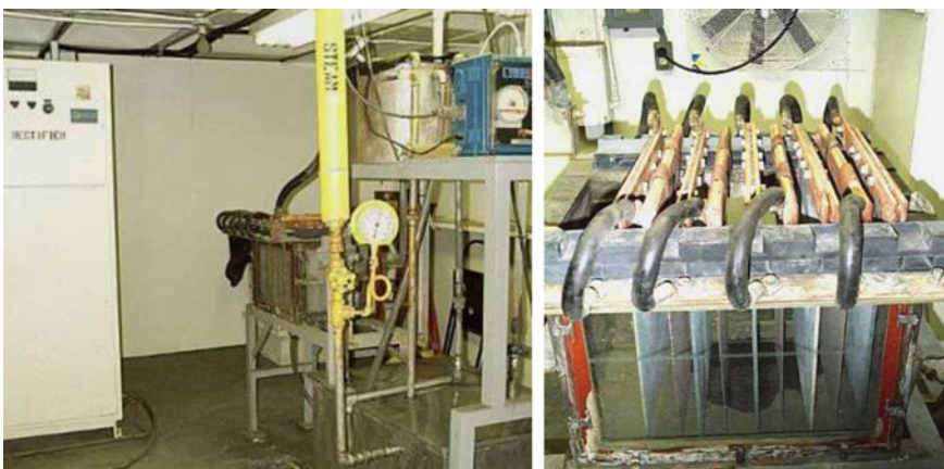
Fig. 2 Copper removal pilot plant and EW test cell. (Color figure online)
