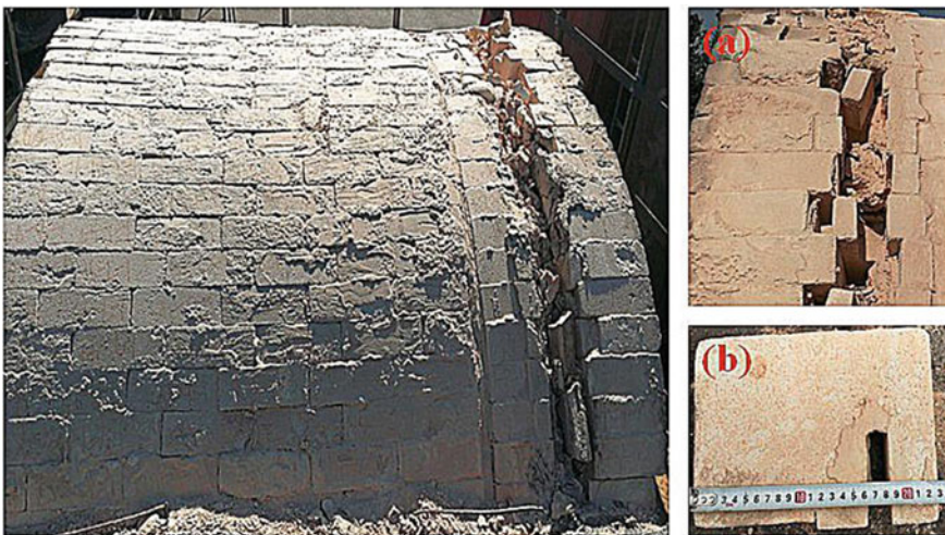
Fig. 3 First ring of clay brick layer. (Color figure online)
