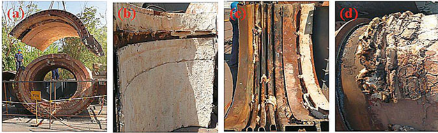
Fig. 2 Disassembly diagram of the upper steel structure of the bellows. (Color figure online)
