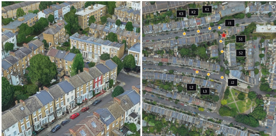
Fig. 5.18 Residential area in London where measurements were carried out and the 1:10 scale model is based on. Study by Salvati and Kolokotroni (2020a), aerial views from Google Earth
