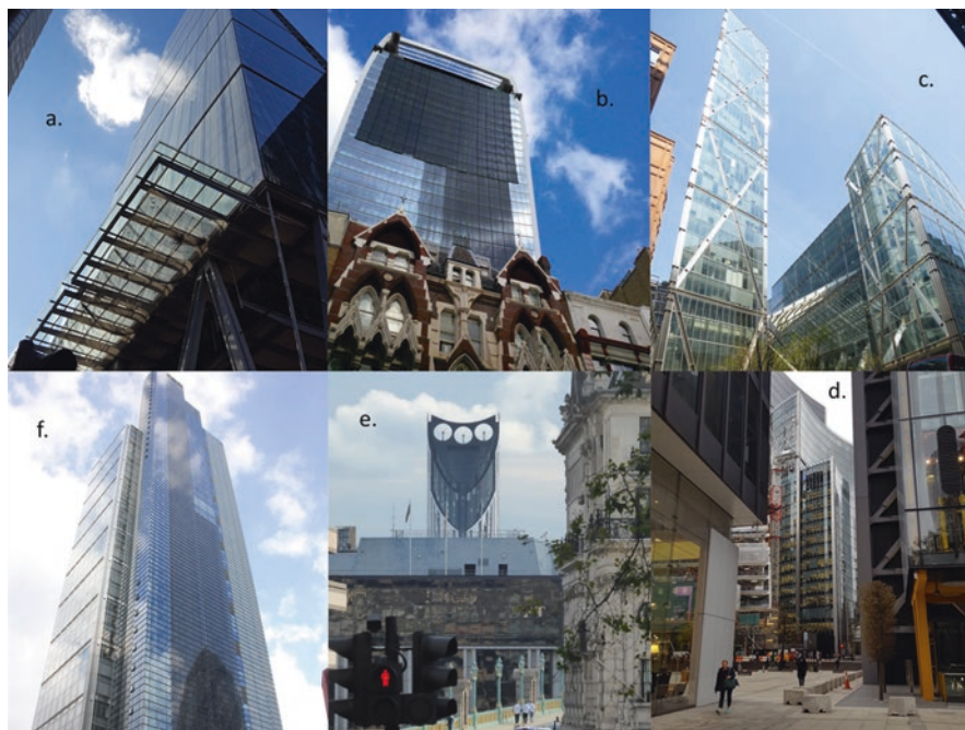
Fig. 9.2 Examples in the City of London that illustrate the relationship between buildings, energy management and outdoor spaces: (a) shows a canopy extension which limits the impact of fast winds that have been displaced downwards toward the ground; (b) shows a covering placed over the south-facing, parabolic shaped glazed façade of a building which redirected and focussed solar radiation onto adjacent streets (the façade was subsequently refurbished); (c) shows a set of tall buildings that channel air through a pedestrianised street and require vegetation to make the space more comfortable; (d) shows a configuration that has a Venturi effect on airflow as it is accelerated through a narrow gap between two very tall buildings; (e) shows a residential apartment block with embedded (stationary) wind turbines that rely on a common resource; and (f) shows a tall structure with embedded photovoltaic cells along its south-facing façade, which has subsequently become overshadowed by a neighbouring building. Each of the buildings shown here is an exemplar of energy-efficient buildings that meet carbon goals (credit: Futcher and Mills)
