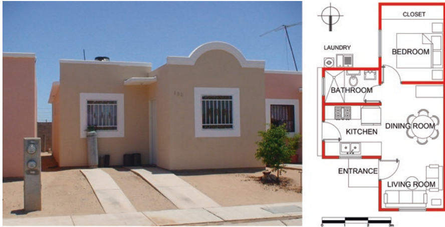
Fig. 8.14 Typical low-cost dwelling constructed in the region (Marincic et al. 2010). View of the façade (left) and floor plan (right)
