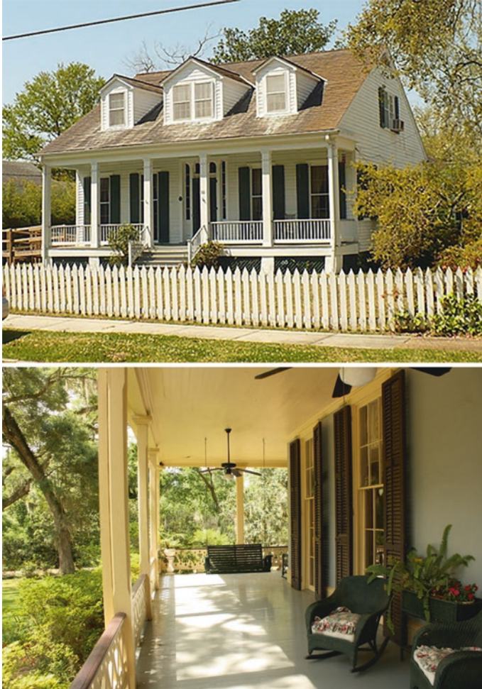
Fig. 7.4 Traditional creole house with shading and terrace (top). Terrace providing outdoor living space and shading of interior spaces (bottom)
